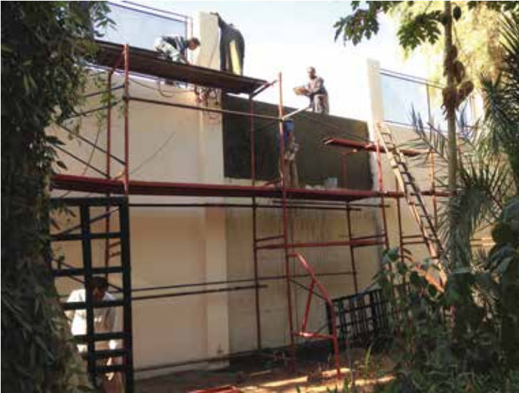
Figure 28. Chicago House southern wall raising (photo: Tina Di Cerbo)
