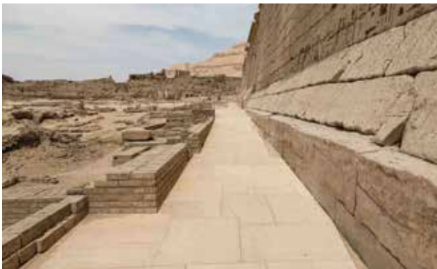
Figure 15. Stone paving and brickwork finished, April 2017 (photo: Ray Johnson)
