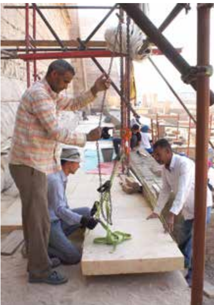
Figure 13. Laying new paving at Medinet Habu, March 29, 2017 (photo: Ray Johnson)
