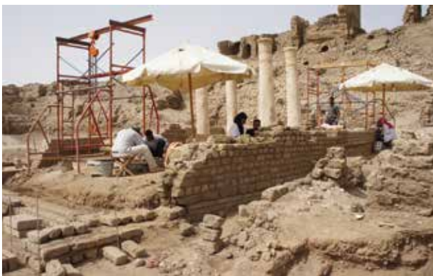
Figure 16. Butehamun House restoration work (photo: Ray Johnson)
