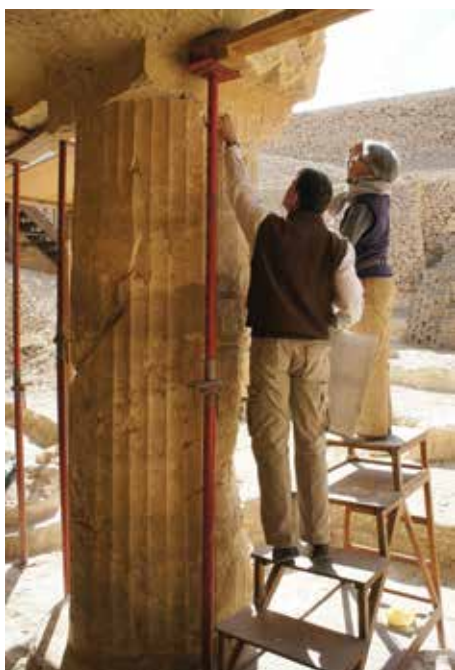
Figure 27. TT 107 Brett and Sue collating pillar, February 3, 2017 (photo: Ray Johnson)
