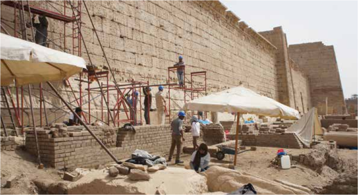
Figure 12. USAID-funded restoration work on southern area M., February 22, 2017 (photo: Ray Johnson)
