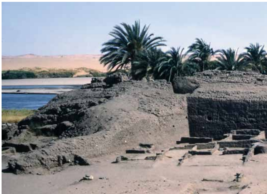
Figure 3. Housing/house units along the north wall at Dorginarti (photo: James E. Knudsta)
