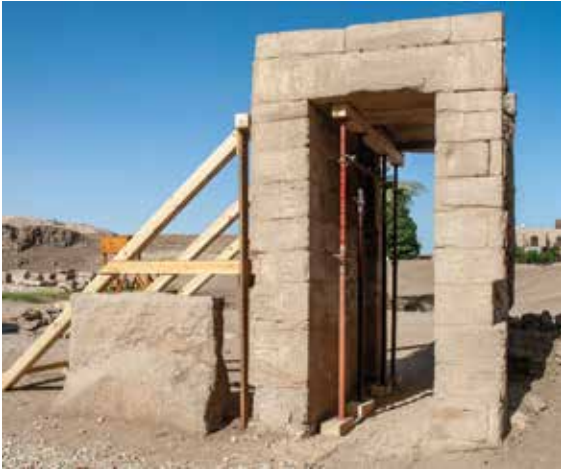
LEFT: Figure 30. Taharqa gate, stabilized prior to dismantling. Photo by Frank Helmholz. RIGHT: Figure 31. Pavement restoration work on south side, west end. Photo by Ray Johnson.
