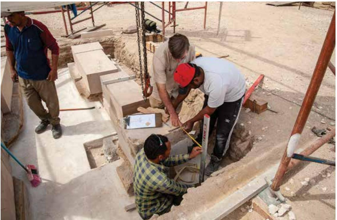
Figure 9. Stonemasonry team reerecting blocks of the Tahrqa Gate. Photo by Mohamed Abo el-Makarem.
