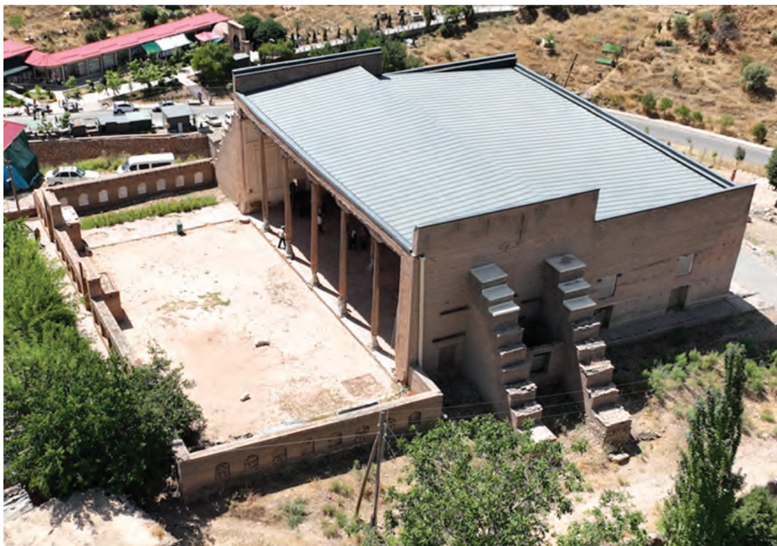
Figure 7. The Langar Ota mosque with its new steel roof, drains, and metal rain caps on the buttresses.
