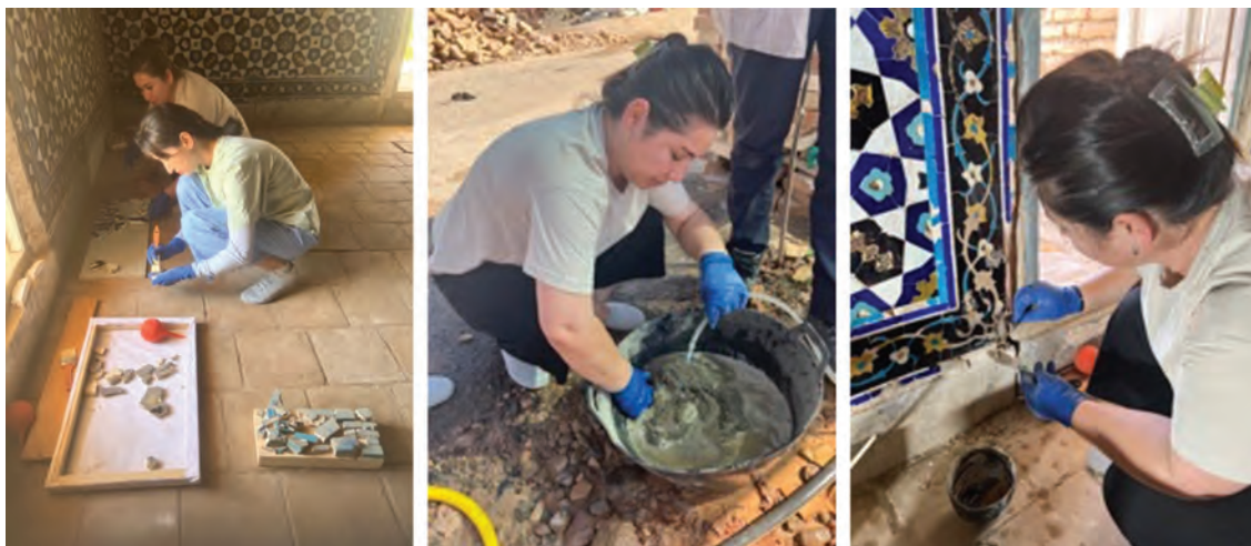
Figure 8. Uzbek conservators Malika Beknazarova cleaning individual cut-tile pieces (left) and Nargiza Kalandarova mixing mortar from traditional building materials and inserting it to repair the geometric tile register (center and right).
