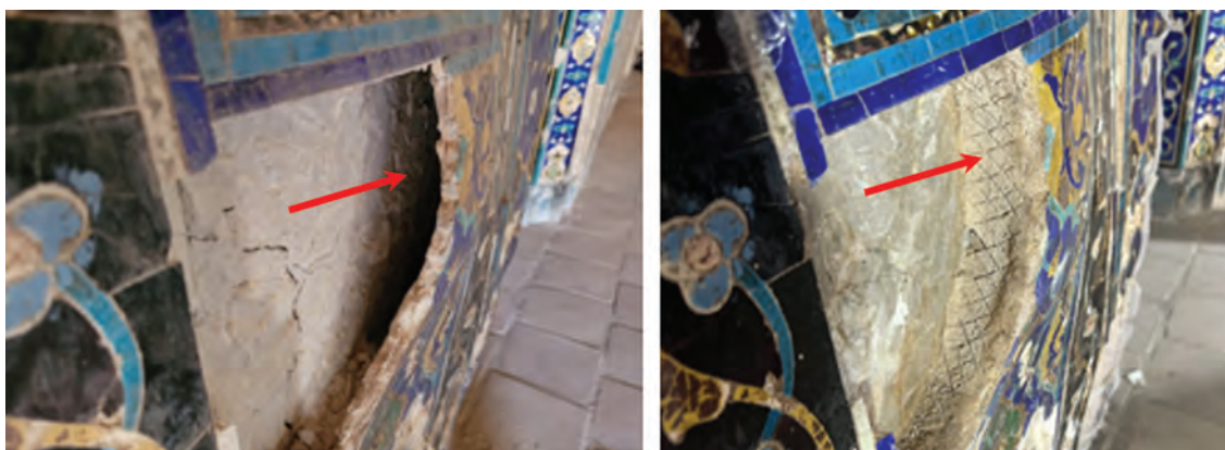
Figure 9. Stabilization of sections of loosened tilework by infilling the voids behind them with sponges soaked in consolidants, then sealing them with mortar made from traditional building materials.
