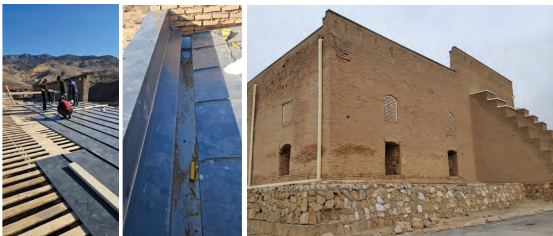
Figure 6. Installation of the new steel roof, steel-sheathed gutters, and drainpipes with extenders to carry water away from the mosque's stone foundations.
