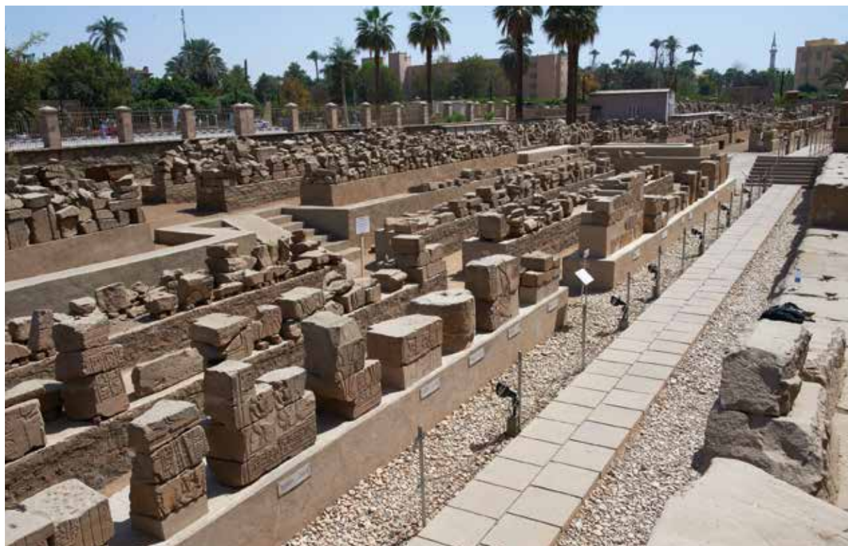
Figure 6.15. The blockyard with mastabas built to store blocks gathered from the Luxor area, 2011. Photo: Y. Kobylecky.
