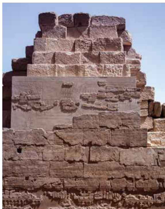
Figure 6.17. Blocks restored to their original location in the upper register of the east wall of the Colonnade Hall, 2005. Photo: Y. Koblylecky.
