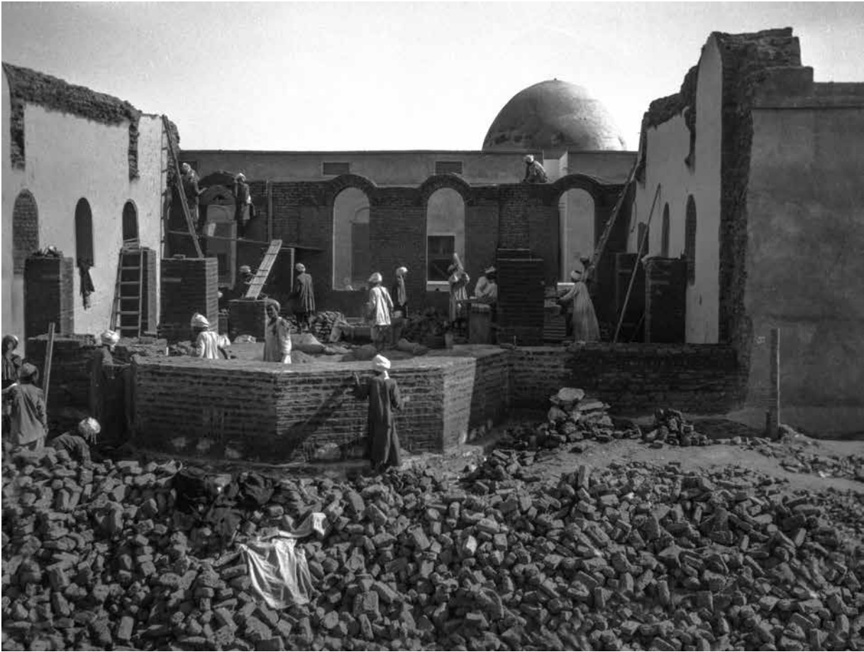
Figure 11.12. Rebuilding of the library when the dome was replaced with a flat roof, January 13, 1927. The dome of the residence is in the background. Photo: C. Ransom Williams, Ransom Williams Collection, Epigraphic Survey.
