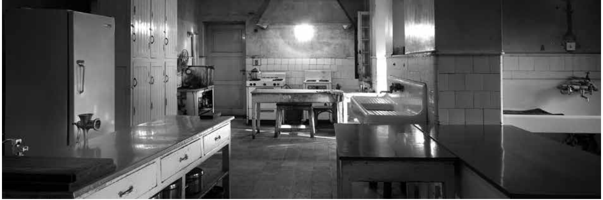
Figure 12.36. The kitchen before renovation, 1991. Photo: T. Van Eynde.
