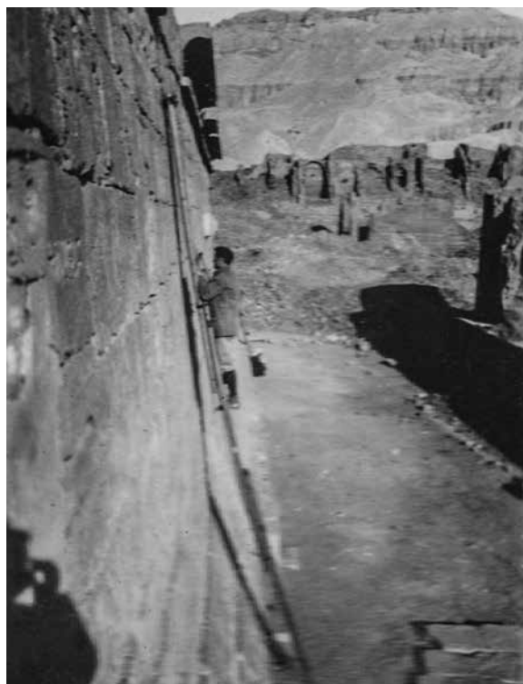
Figure 3.6. Alfred Bollacher working on a tall ladder on the north wall of Medinet Habu, ca. 1930. Photo: E. DeLoach, Chubb Collection, Epigraphic Survey.
