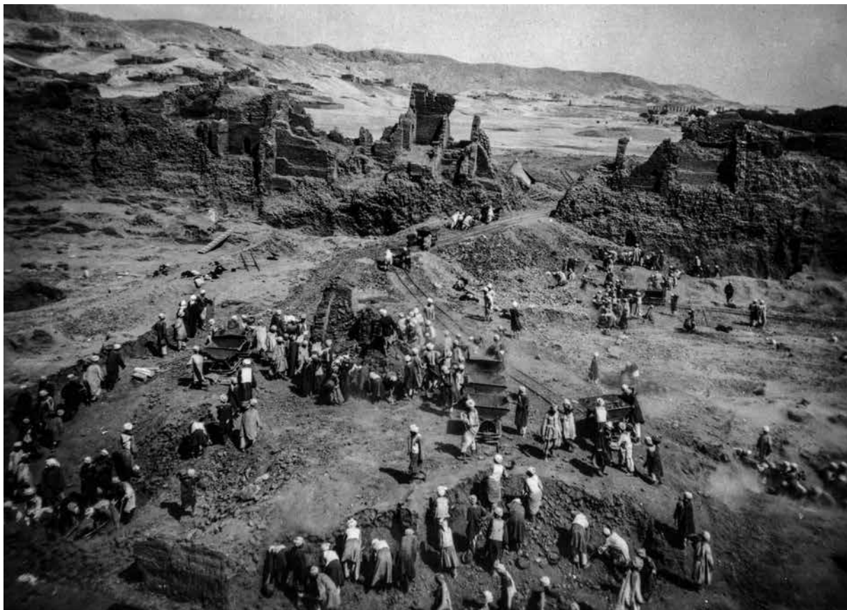
Figure 4.4. Excavation in progress, with railway used to remove debris, ca. 1929. Photo: Epigraphic Survey.
