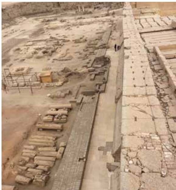
Figure 3.55. New mudbricks, stamped with “UC,” used to cap and protect the ancient walls (left), April 2017. Photo: F. Helmholz.
