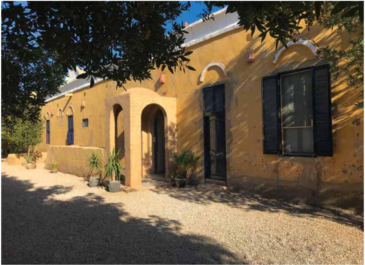
Figure 11.24. The Marsam Hotel, which incorporates part of the original Chicago House. Photo: E. Teeter.
