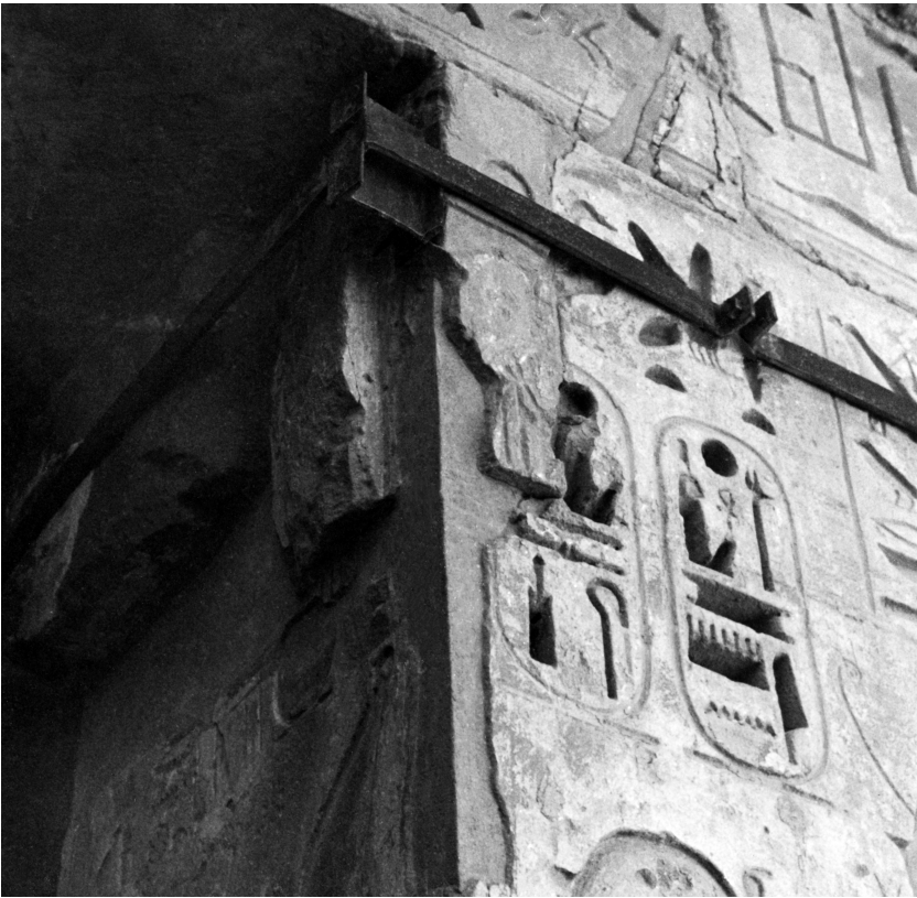
Fig. 3. Outer corner of pillar showing later patch stones; compare pl. 218. Photograph by McClain.
