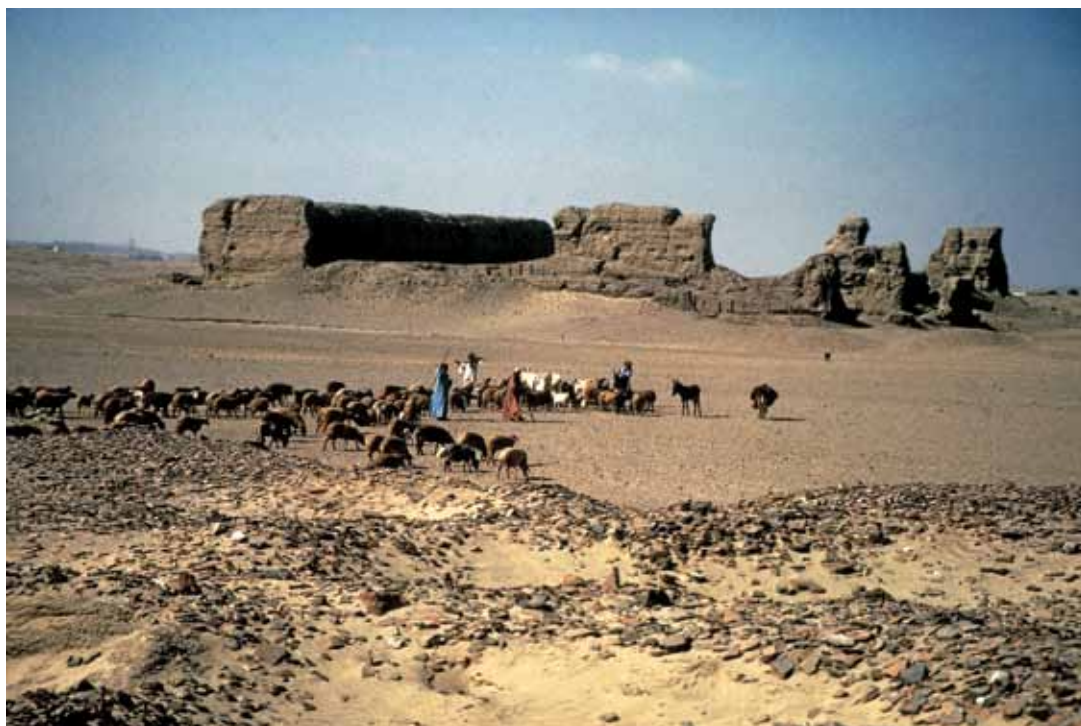
FIGURE 4.20. The "Fort," the ceremonial enclosure of King Khasekhemwy of Dynasty 2, the oldest freestanding mudbrick structure in the world
