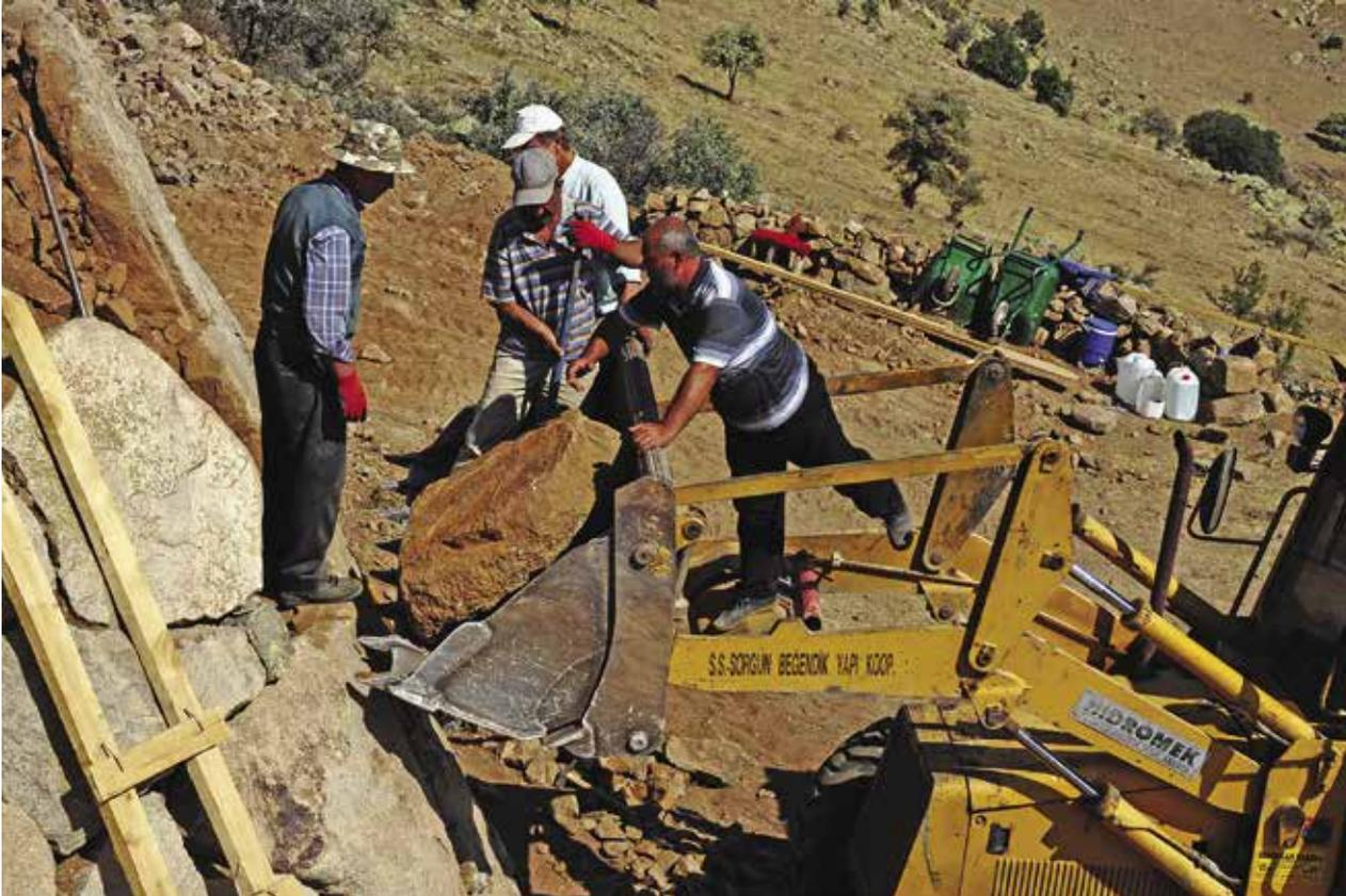
(b) A mechanical excavator with a backhoe and front bucket was used both as a lift or crane to haul and raise the building stones and as movable scaffolding for the masons.
