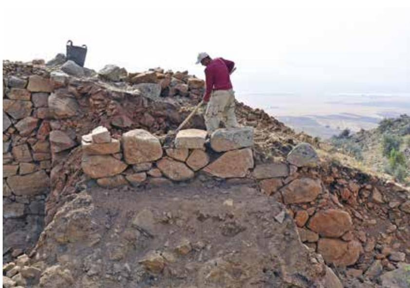
(c) Restoration of the glacis was essential if the very loose fill of rubble and soil was to be stopped from washing down.
