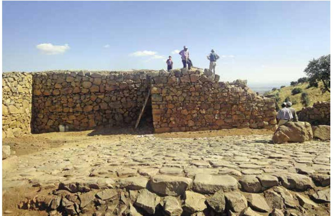
(a) The northern face of the Middle Tower was rebuilt according to the survey and documentation project during the 2011 season. However, as horizontal timber beams were not used, this part collapsed after heavy rains.
