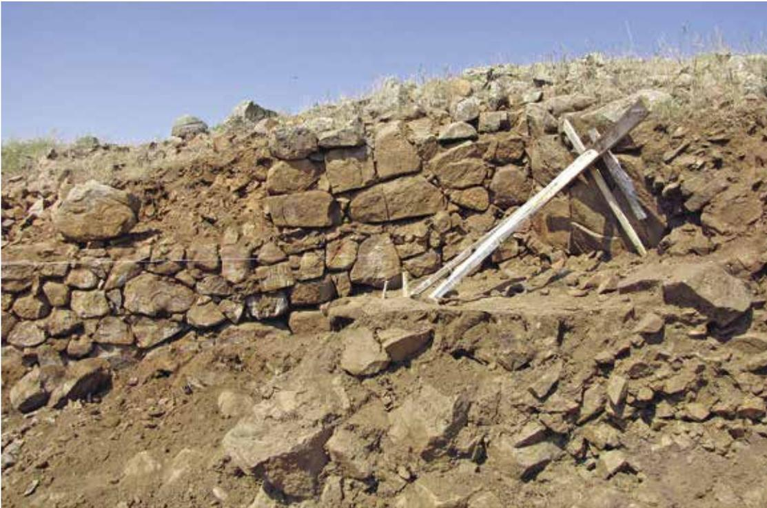
(a) The loss of horizontal timber beams due to fire or deterioration has led to the dislocation of the face stones and created wall surfaces that incline outward.
