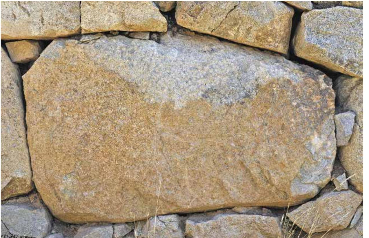
(b) Face stone in the northeastern wall of the passage showing pecking marks where trimmed |
