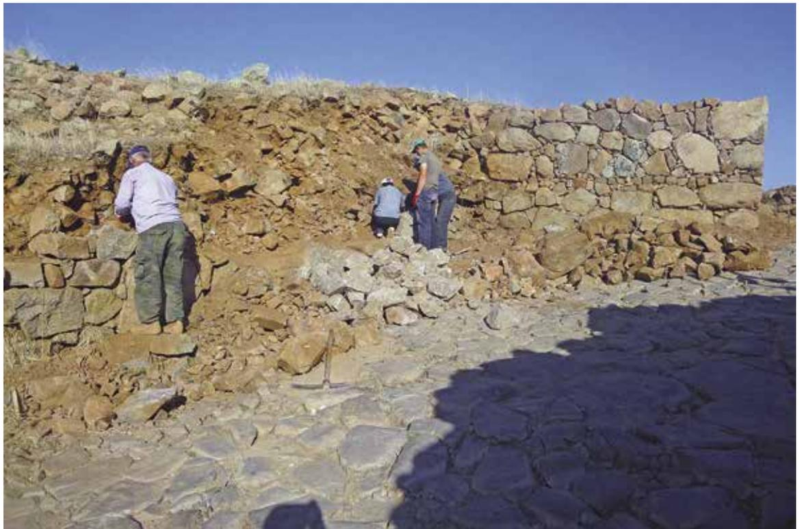
(b) The southern face of the West Tower completed and the western wall of the front gate passage being cleared of fallen debris before the building of a temporary retaining wall
