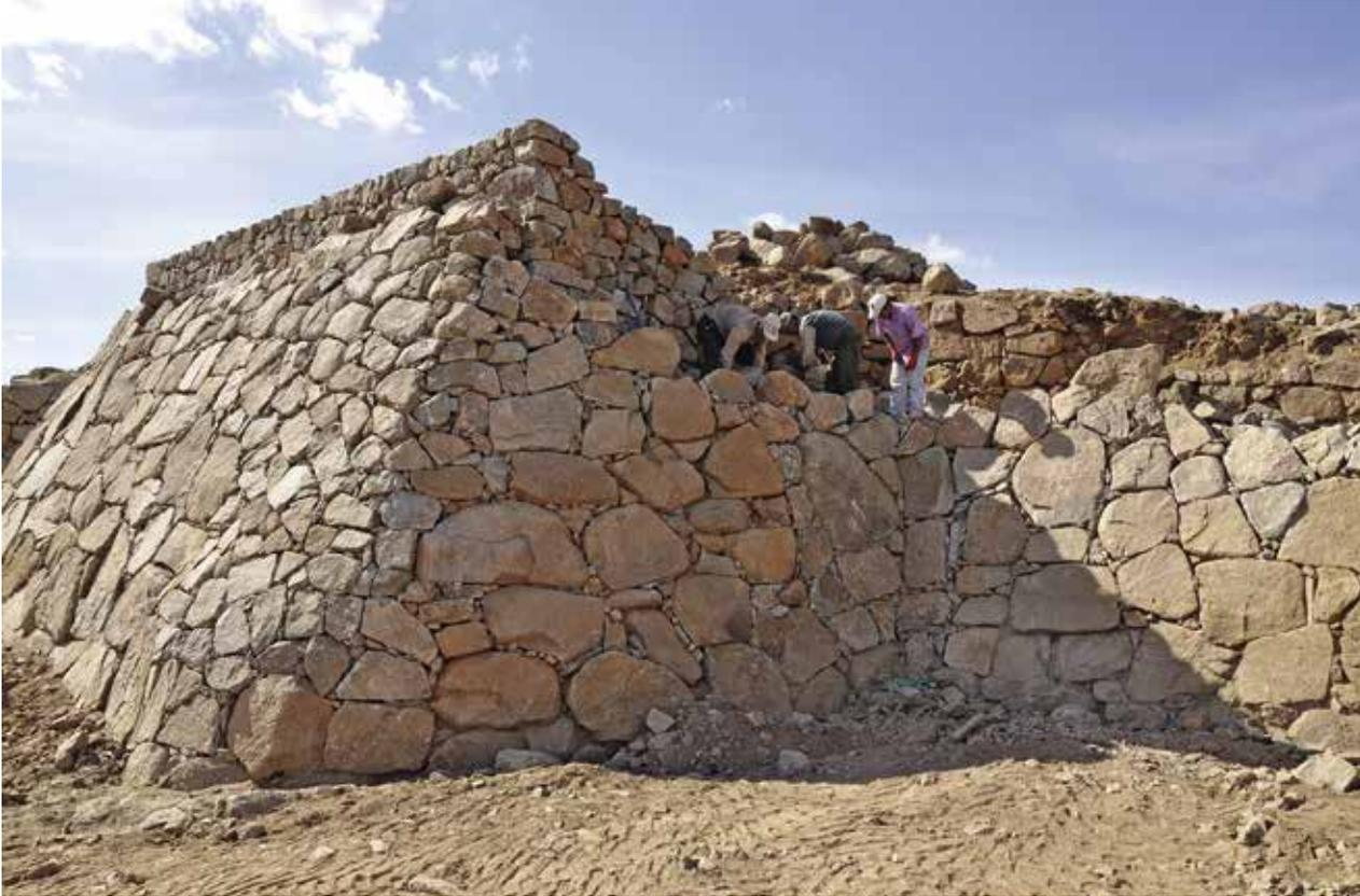
(a) The southeastern corner of the East Tower was rebuilt with comparatively smaller stones that can be distinguished from original work.
