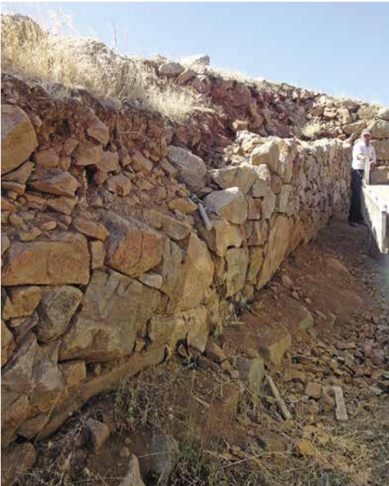
(b) The western side of the front passage adjoining the southern face of the West Tower was rebuilt to function as a temporary retaining wall against the infill that was likely to have washed down on to the gate court pavement otherwise.
