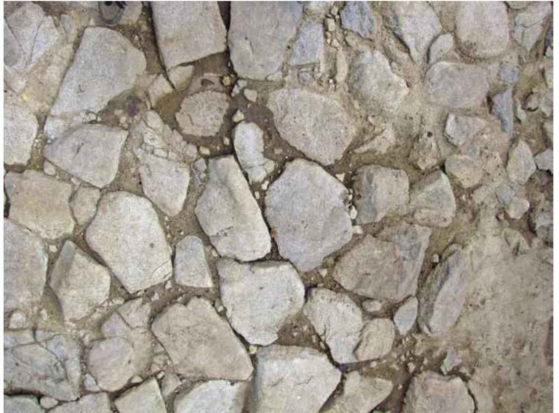
(a) The slightly sunken stone in the center of the entrance passage after rain. Marks toward the upper left and lower right are 1 m apart. |
