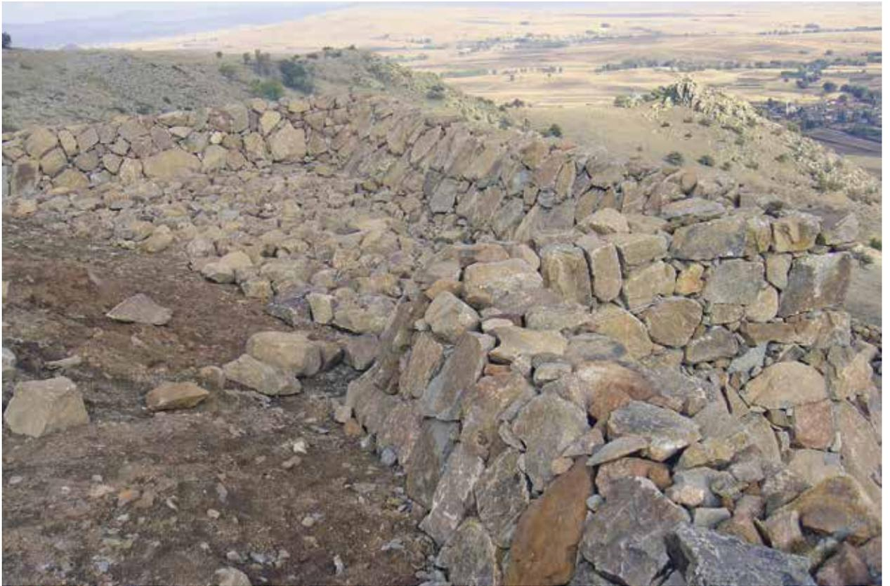
(a) As a safety measure, the restored tower walls were raised to form a parapet to prevent visitors from walking too near the edge. |
