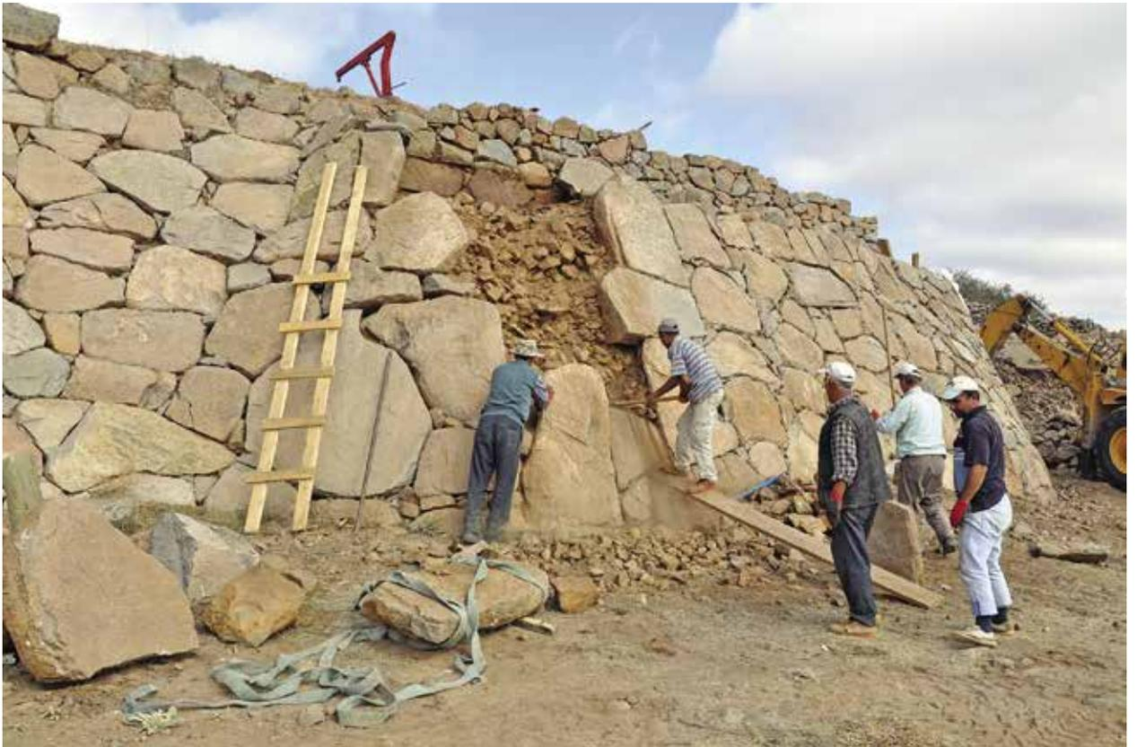
(b) Once the eastern side of the glacis was built up to the height of the adjacent stretch of glacis, it was found necessary to relocate two slipped stones before rebuilding the top of the glacis. |
