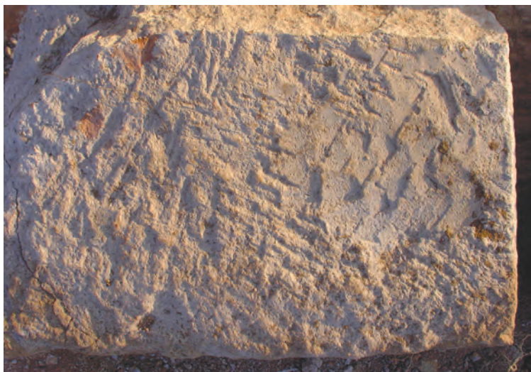
| (c) Coarse toolmarks left by a broad chisel and a point
