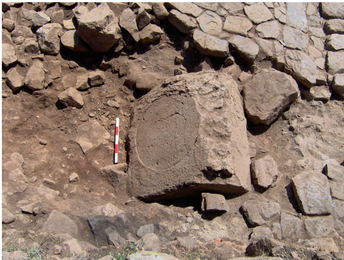
(a) Column base in rear section of the Monumental Entrance, tilted by treasure seekers who burrowed underneath it, with part of damaged drain at right
