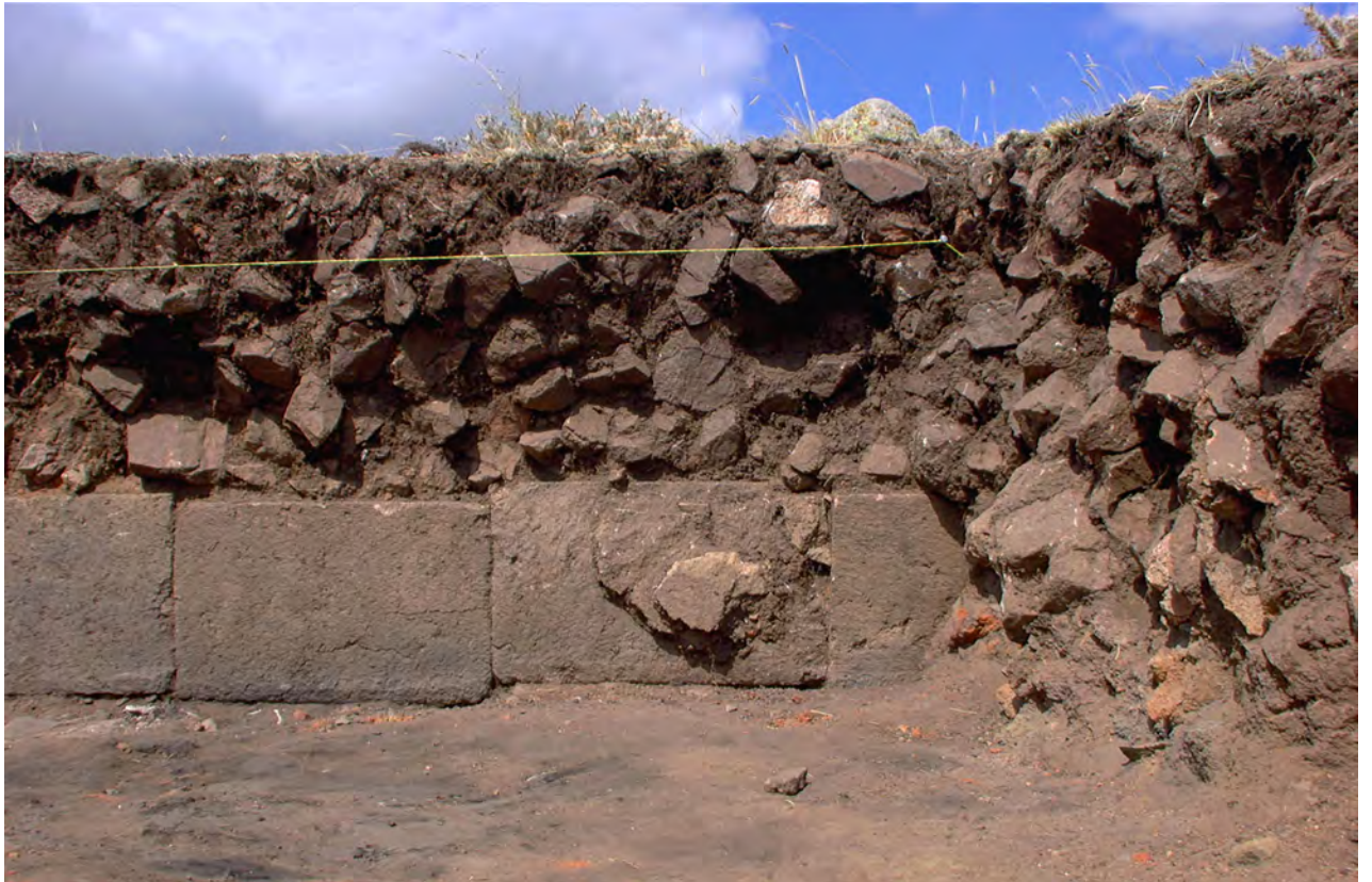
(a) Ashlars 30-32, in western wall of the Ashlar Building, with fallen mud plaster adhering to ashlar 31 |
