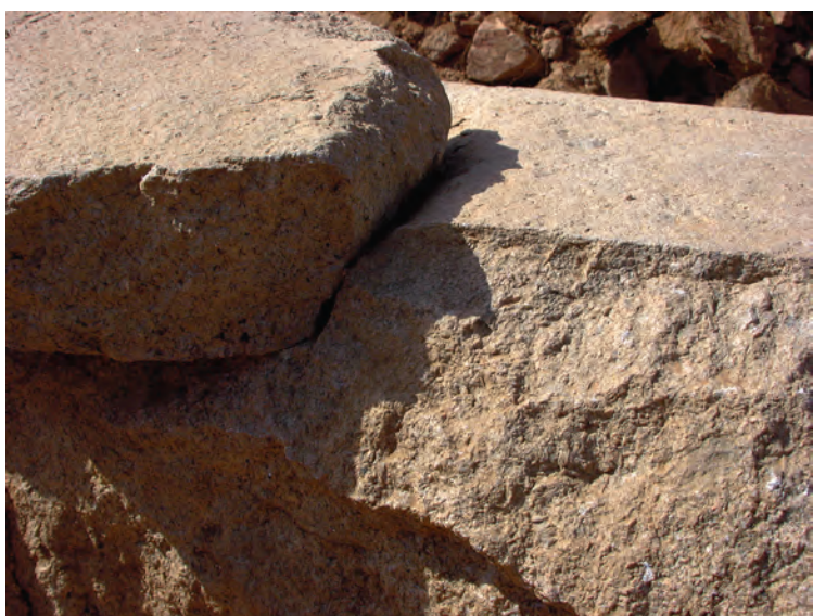
(c) Detail of fitted granite in southern wall of the North Platform where wall front has broken away
