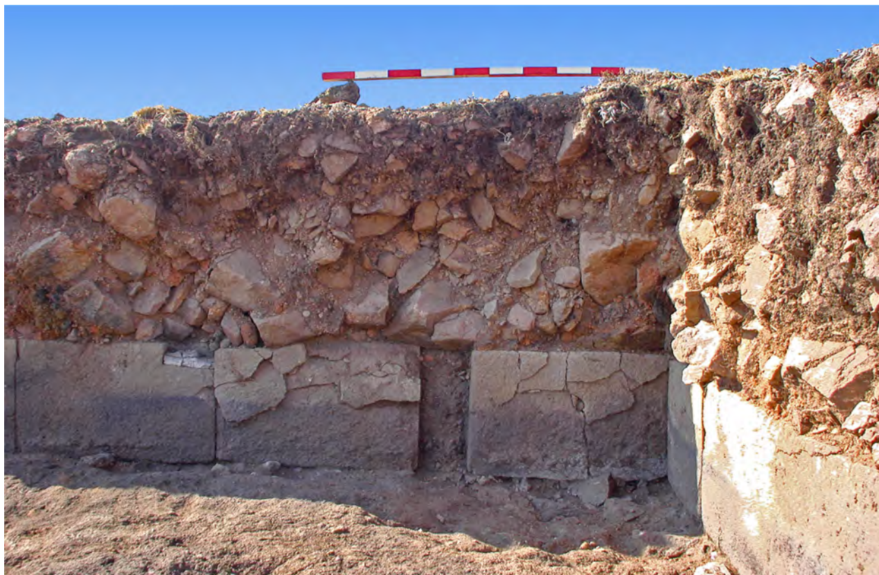
| (a) Western end of southern wall of Room 2 showing limestone plug at top left corner of ashlar 24 (at left) and gap between ashlars 25 and 26
