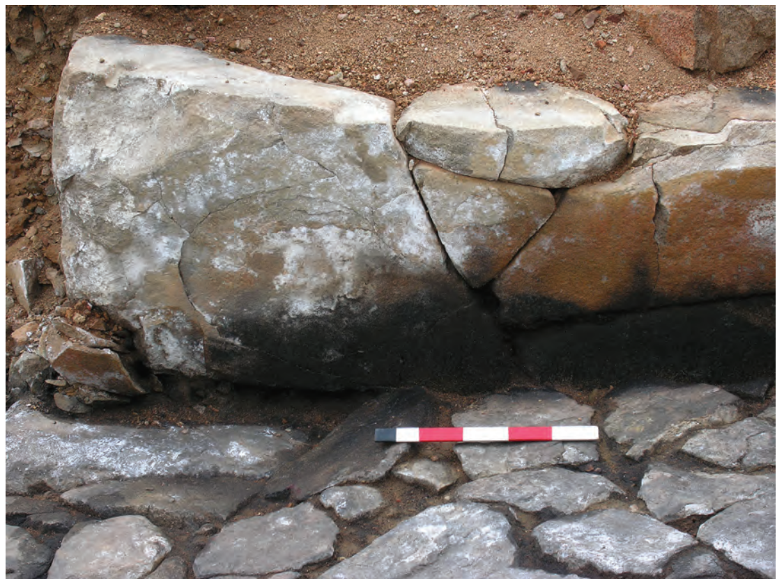
(b) Granite, shaped to fit tightly between two large blocks in northern wall of the South Platform, showing fire damage |
