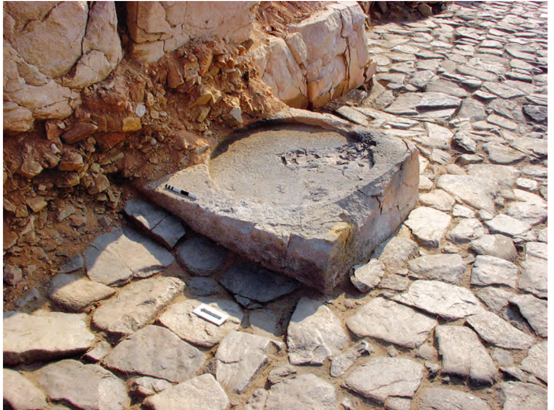
(α) Northern column base, before total removal of burned debris, showing very severe damage caused by fire. The scale is 20 cm. |
