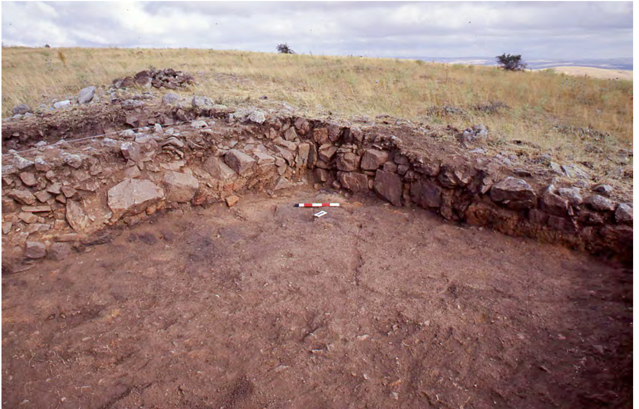
(a) Northeastern corner of the Audience Hall in TT22 showing poor condition of the walling |
