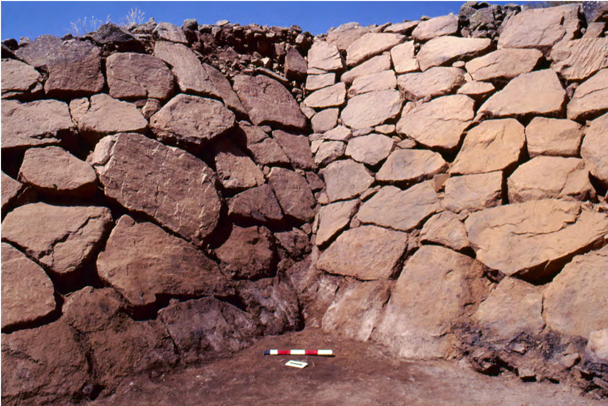
(a) Sharp corner of Structure A glacis around South Tower and the recess showing how the face stones are bonded. Hard black mineral accretions on the glacis face can be seen at lower right. The 50 cm scale rests on the clean surface that is probably mud plaster washed down from the wall face.
