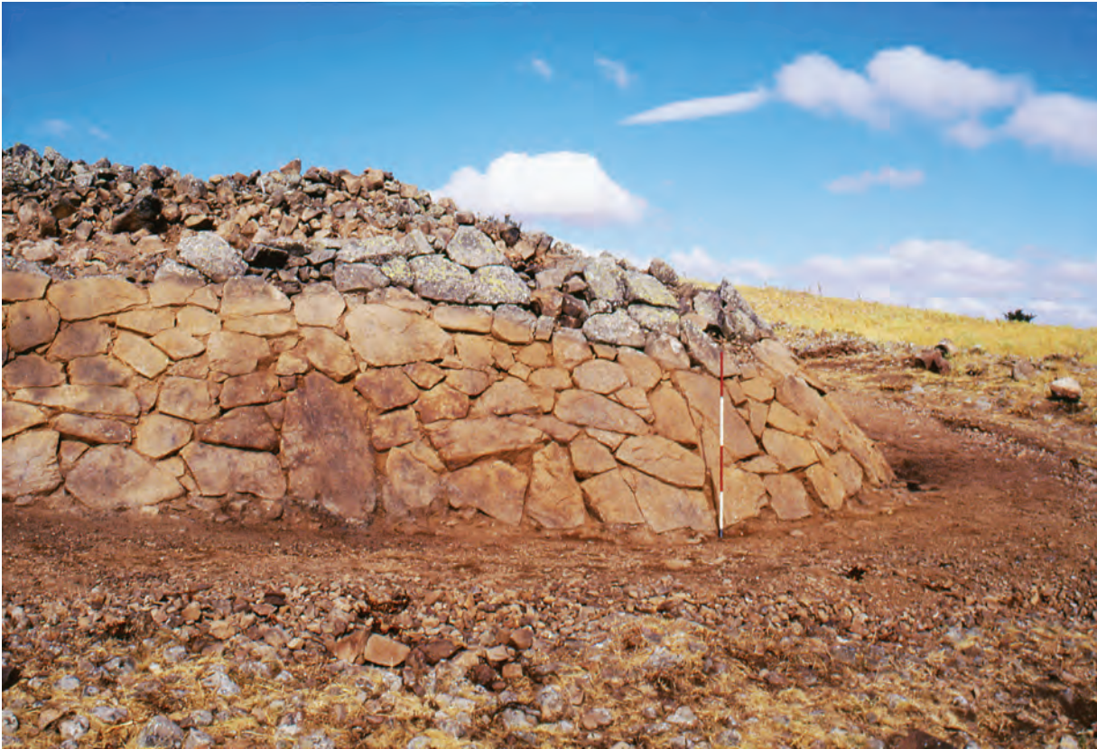
| (a) Structure A glacis around northeastern corner of North Tower
