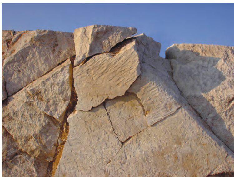
| (b) Faced block of fine, very pale brown sandstone with toolmarks in different directions
