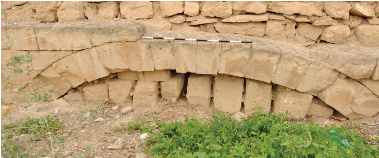
Figure 6.17. Sunken arch (“water gate”) in the western enclosure wall, opened apparently at the point where the bed of a dry stream crossed the line of the wall, running afterward between the two main buildings (the qaṣr and the Audience Hall) through the open space left between them. The location of this water gate is circled in red on the plan in figure 6.16d.
