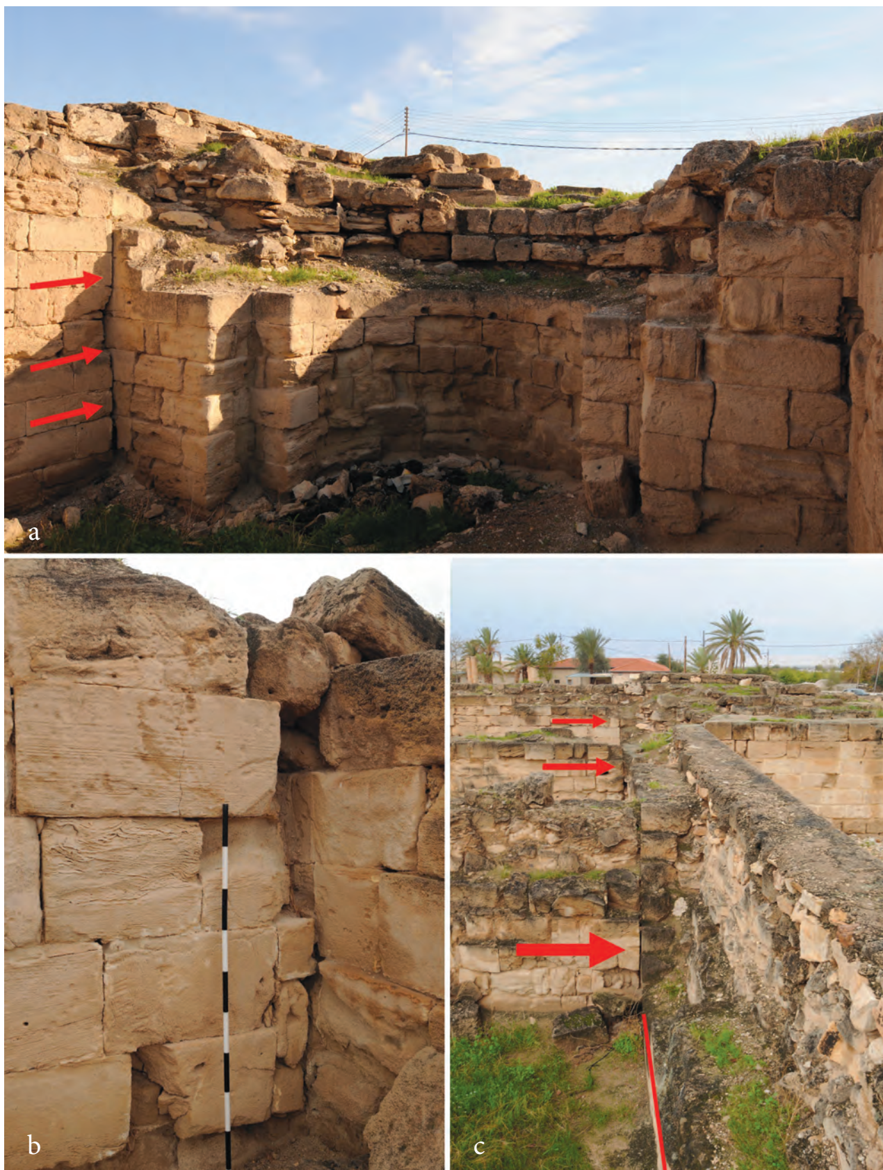
Figure 6.3. First congregational mosque within the palace ( qaṣr ). a , View of the miḥrāb . Note the disproportion between its span and the width of the prayer hall, as well as how the late partition walls abut the qibla wall. b , Later partition walls abutting the end pilasters of the north wall of the original first congregational mosque. c , Later partition walls abutting the qibla wall and dividing the space of the original mosque.
