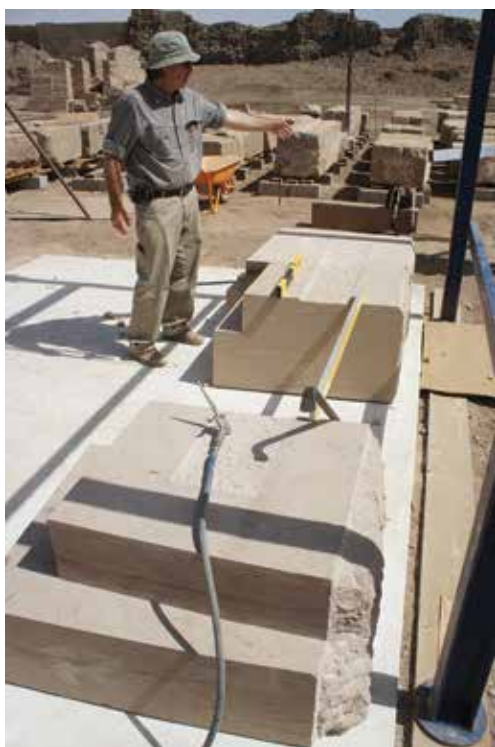
Figure 9. Frank and new Domitian Gate footing March, 2013 (photo by Ray Johnson)
