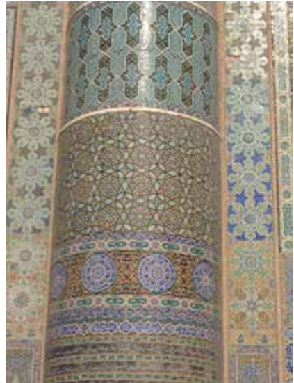
Figure 12. Detail of some of the glazed tile work on the Masjid-i-Jami in Herat
