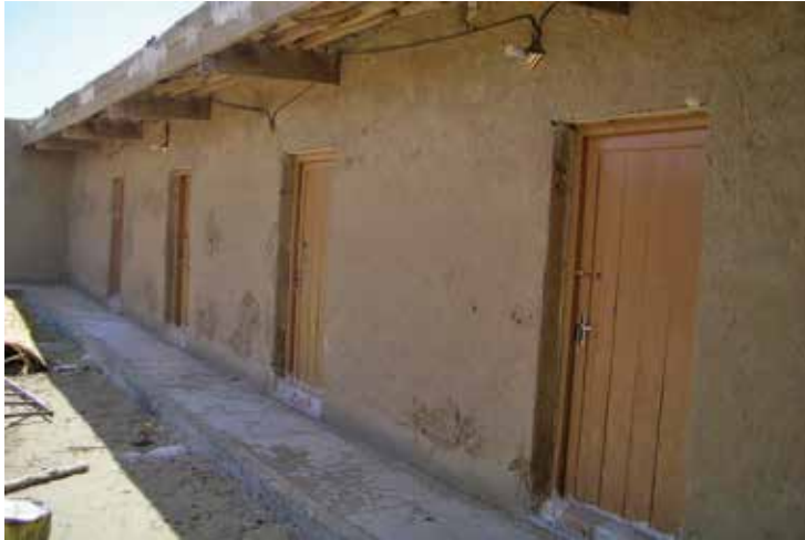
Bedrooms with restored doors
