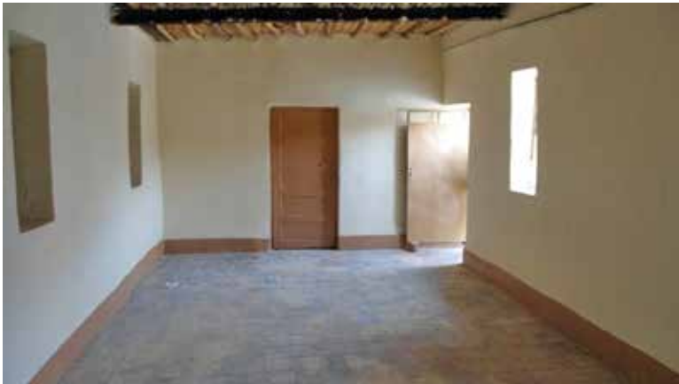
Workroom painted during house repair, May 2015
