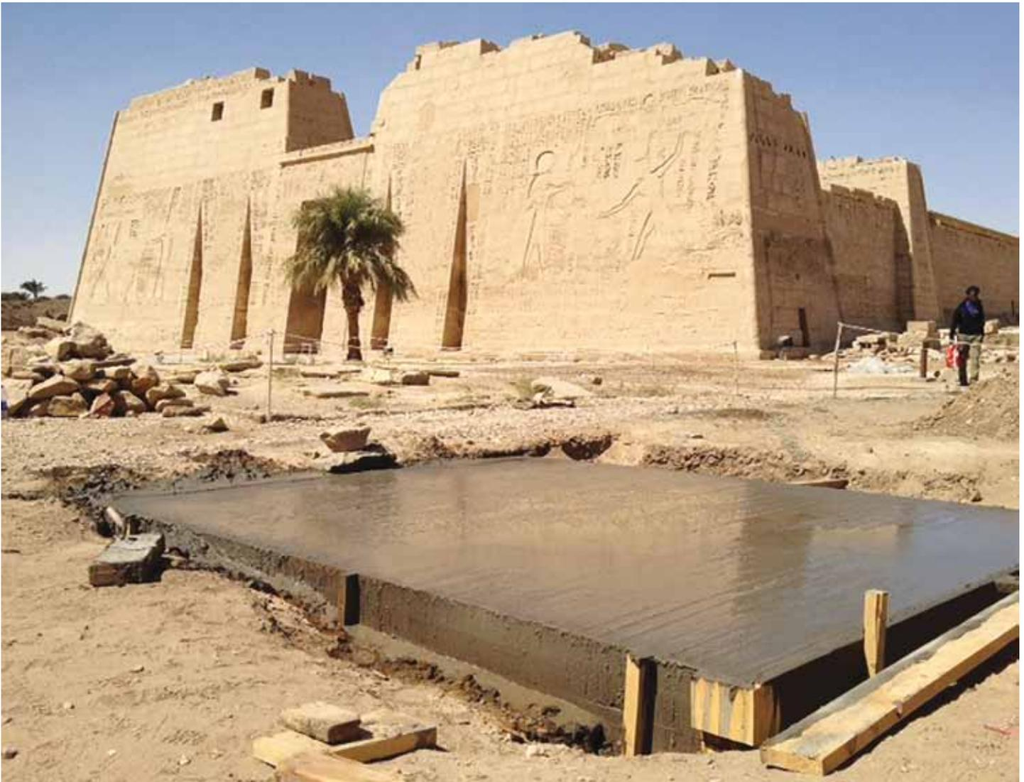
*Poured, reinforced-concrete foundation for the Domitian gate. Medinet Habu (photo by Frank Helmholz)*
