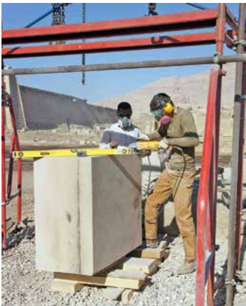
Left: Saber and Johannes smoothing and finishing a block. Right: Domitian Gate block erecting. Photos by Ray Johnson
