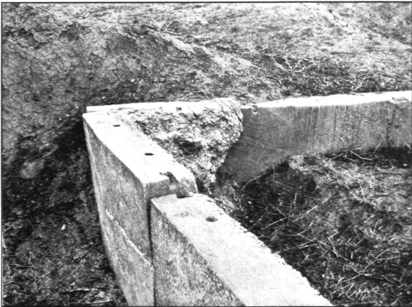
FIG. 61. CORNER OF ROOM IN PALACE OF ASHUR-NASIR-APAL. Note the use of the dowel holes.
