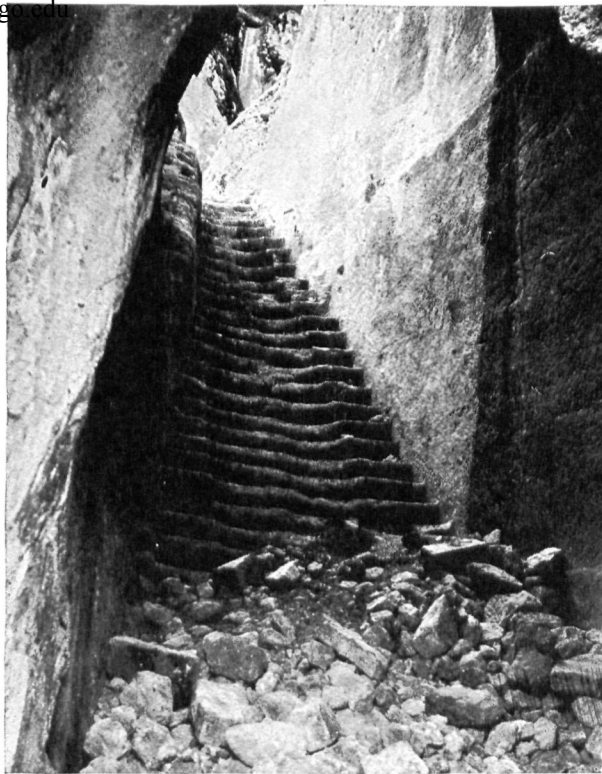
FIG. 172. UNDERGROUND STAIRS. (Fort in Asia Minor.)
