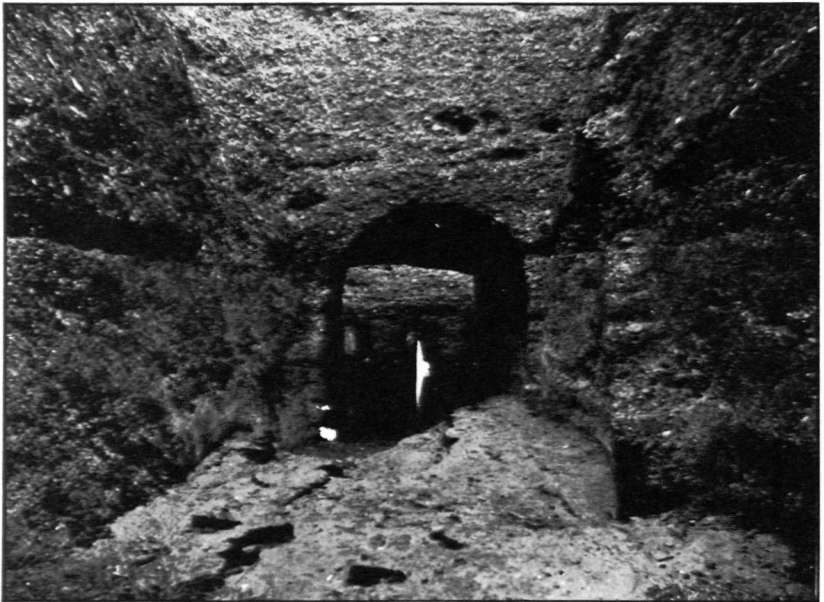
FIG. 144. WATERWORKS AT NEGUB, BUILT BY ASHUR-NASIR-APAL AND RESTORED BY ESARHADDON.
