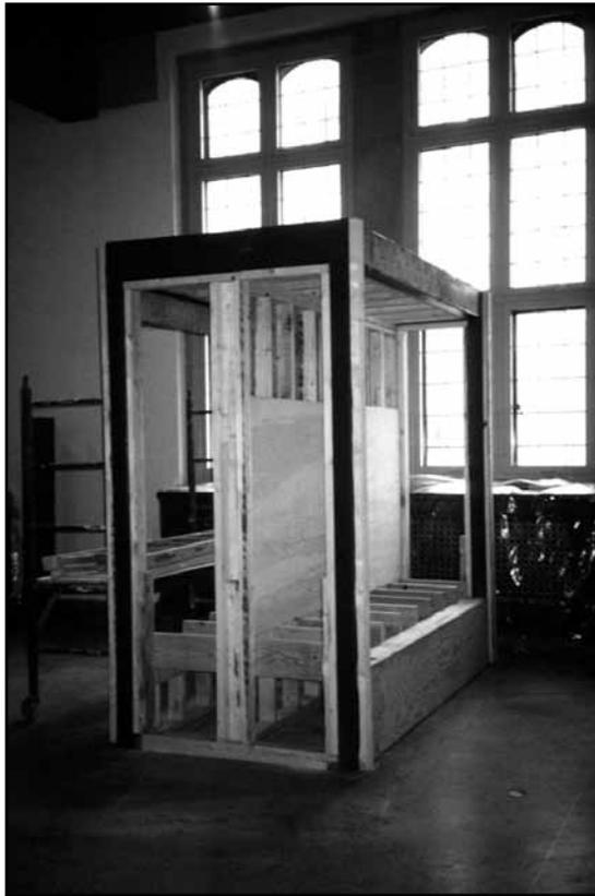
***Carpenters frame steel in wood and build central divider for this case to produce two separate exhibit areas. New cases are constructed over welded steel framework that is bolted into gallery floor***
