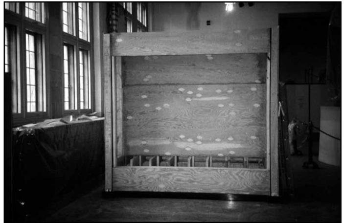
***View of west side of new exhibit case that will feature heavy funerary reliefs; at this stage of construction, reinforced deck and space for recessed lights are prepared***
