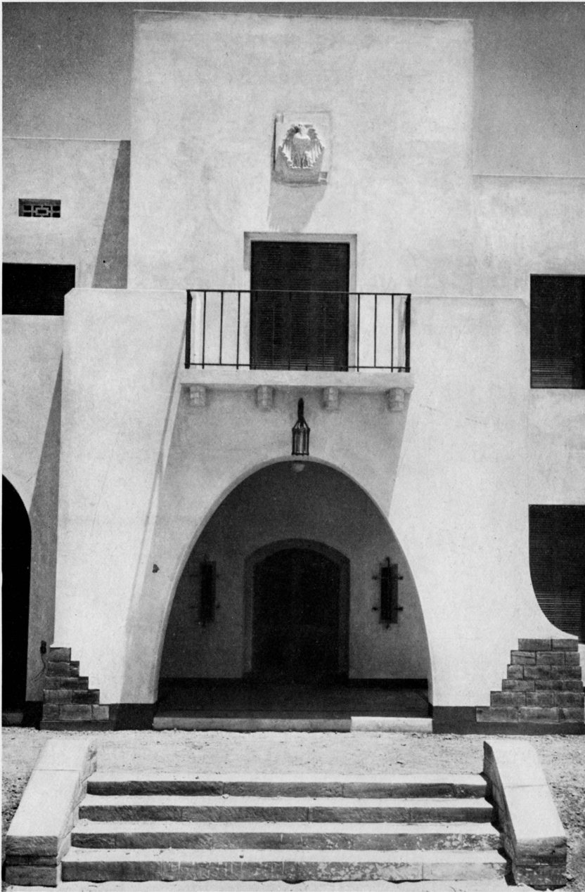
FIG. 24.—THE NEW HEADQUARTERS AT LUXOR. MAIN ENTRANCE OF THE RESIDENCE BUILDING
