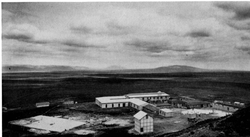
FIG. 50.—HEADQUARTERS BUILDINGS OF THE PALESTINE EXPEDITION OF THE ORIENTAL INSTITUTE AT ARMAGEDDON (MEGIDDO)
