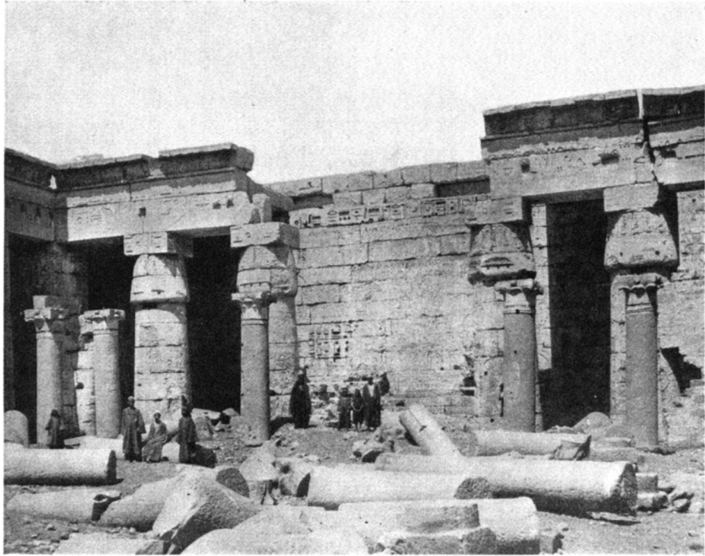
FIG. 35.—REMAINS OF COPTIC CHURCH WHICH STOOD IN SECOND COURT OF THE GREAT TEMPLE, AS SEEN BEFORE 1891, THE YEAR IN WHICH THAT COURT WAS CLEARED
