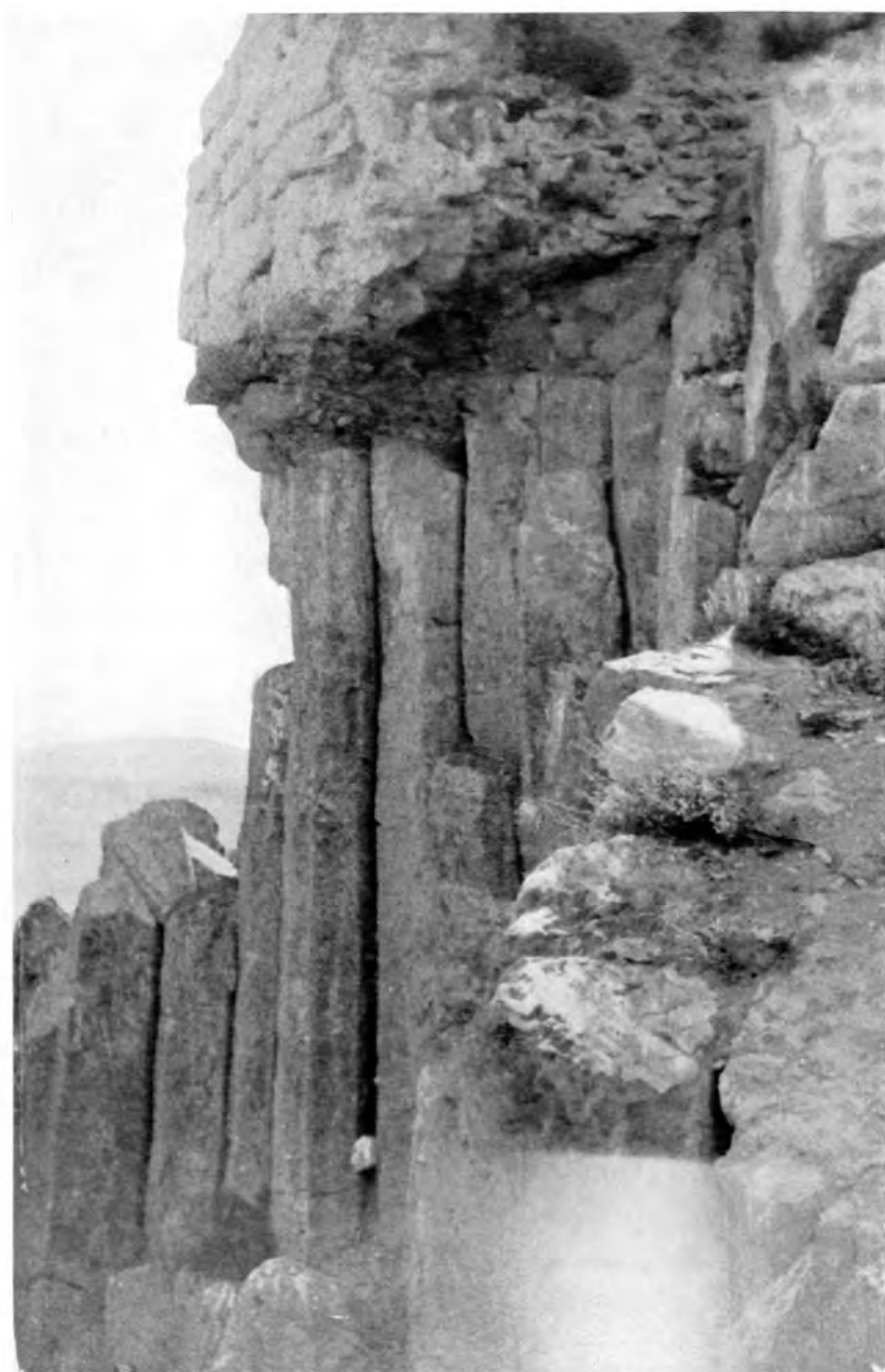
FIG. 105.—Musalim-Kale. Base of wall resting on mass of columnar basalt
