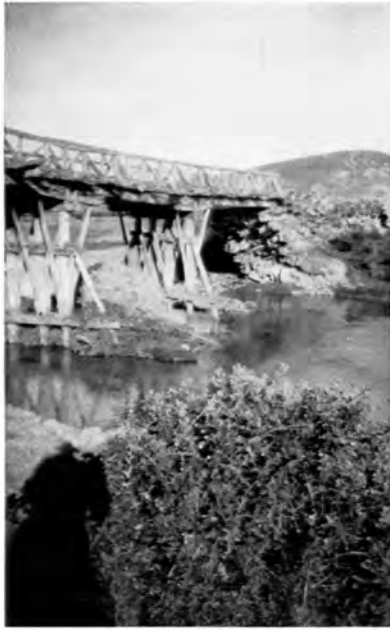
FIG. 103.—Kesik-Köprü. Modern wooden bridge carried on remains of ancient masonry.
