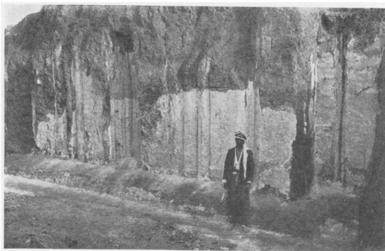
FIG. 92.—Portion of outer wall of the Nabu temple
