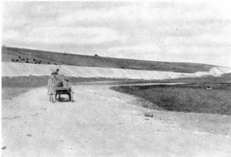
FIG. 56.—The new railroad track from Samsun to Sivas
