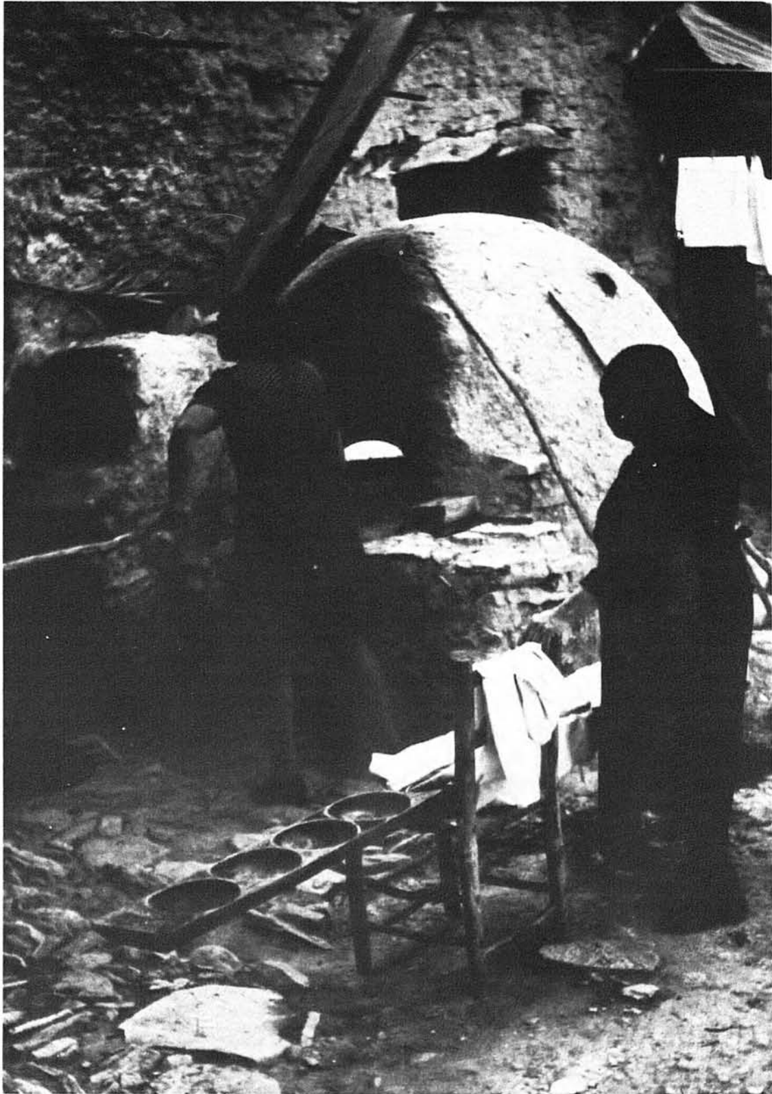
Compound 70. View of the southwest corner, looking northwest from a southern entry room, during the activity of bread baking. Several of the objects being used in this scene can be located at rest in plate 1.
