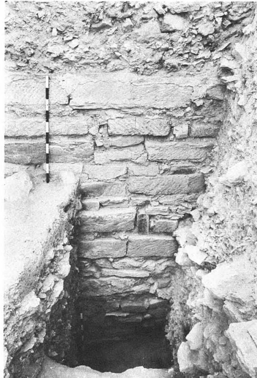
c. East face of Wall 021. Robbed out sandstone courses above top of meter stick. Below robber trench, courses of tabular limestone with diagonal chisel marks. Upper course has "tuck pointing" of gypsum mortar.
