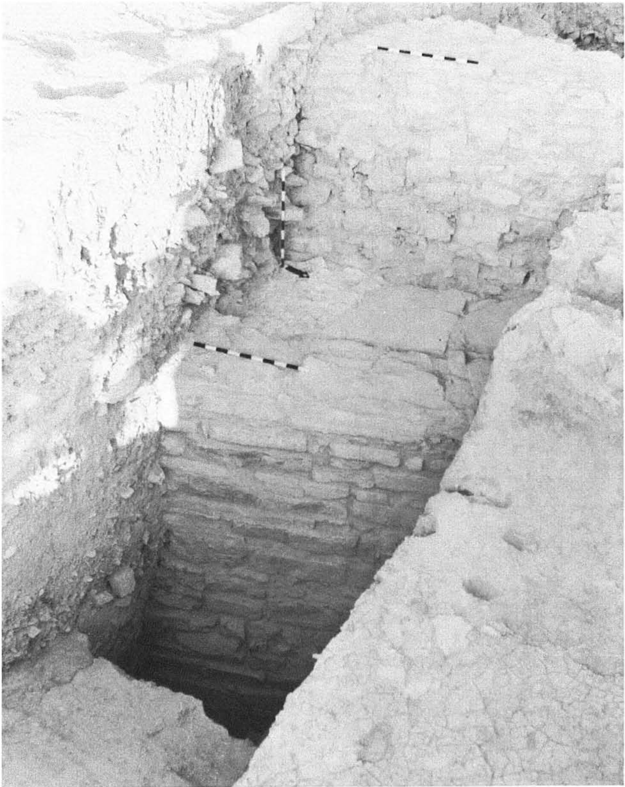
East Face of Citadel Wall 021. North arrow rests on remnants of ashlar sandstone interior face (robbed out), behind which lies core of small limestone boulders and rubble fill.
