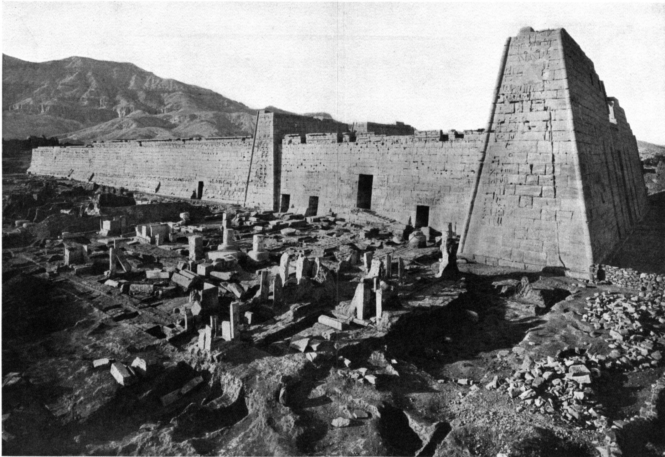
FIG. 28.—GENERAL VIEW OF THE PALACE OF RAMSES III AT MEDINET HABU AFTER EXCAVATION
