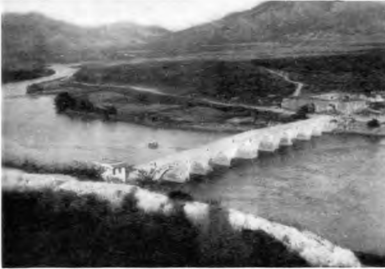
FIG. 58.—The bridge over the Jeyhan at Misis
