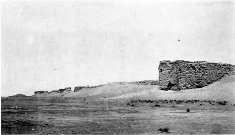
1.—Looking Northwest along Southwest Wall: Southwest Gate near Middle (Pl. I, 2) Seen on Right. Note Sand Drifts Rising to Crest of Wall in Places.
