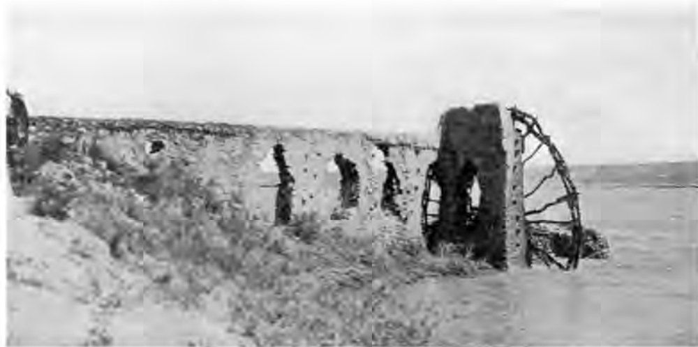
FIG. 9.—IRRIGATION WATER WHEEL IN THE EUPHRATES AT ḤADĪTHAH
