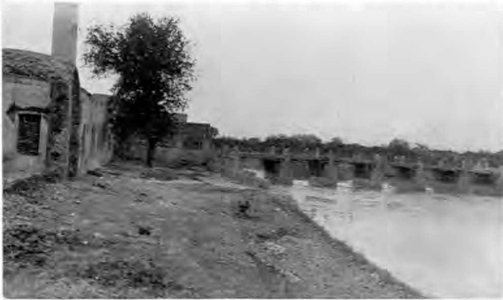
FIG. 22.—THE BRIDGE AT DEIR EZ-ZŌR
