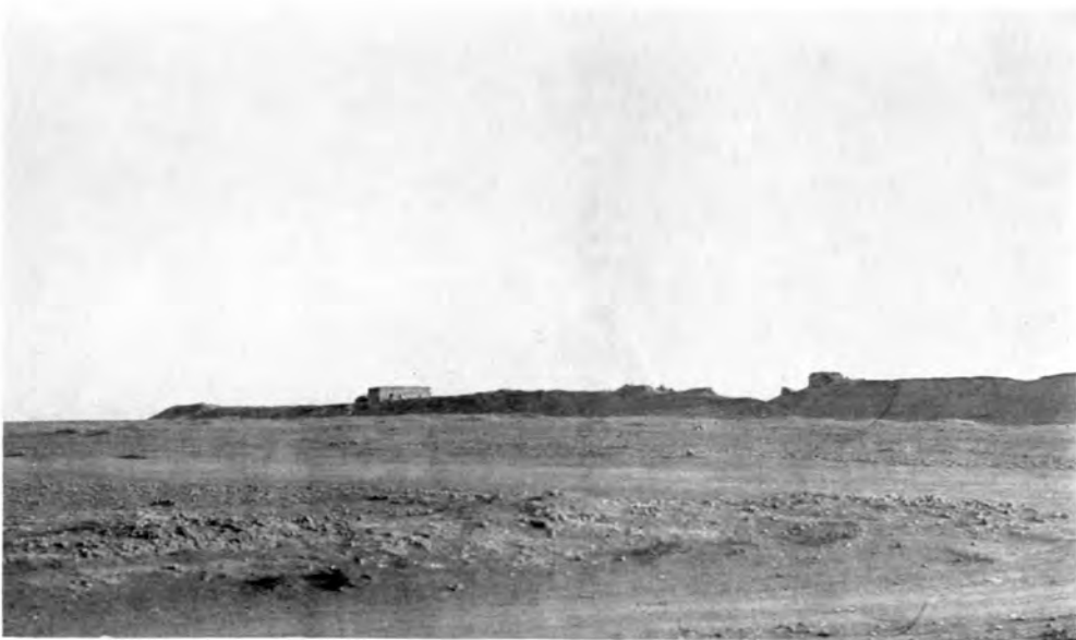
2.—View along Inside of Same Wall. Looking Southeast past Inside of Southwest Gate. Note Sand Drifts Rising to Crest of Wall in Places.
