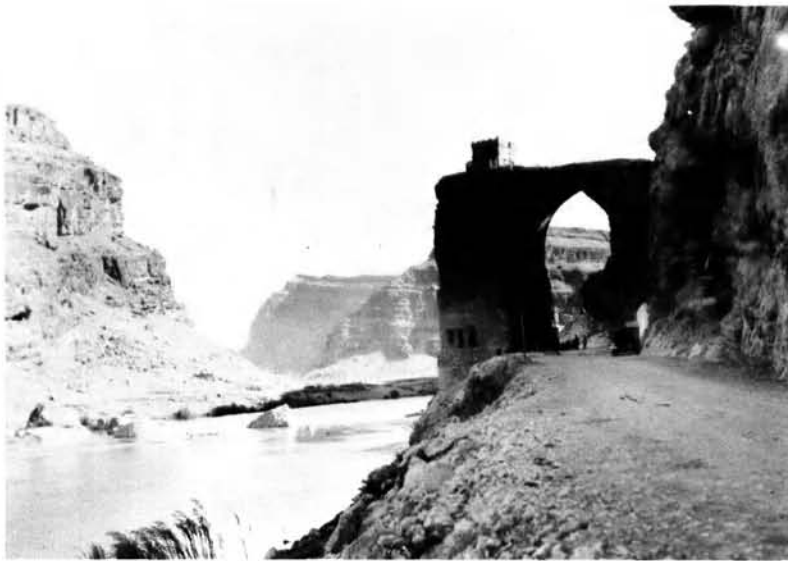
(c) Pul-i-Dukhtar, Kashgan Rud. Bridge (View from South).
