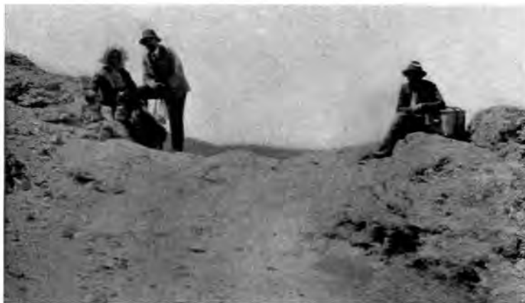
FIG. 105.—KESKIN SIVRISSI. ROADWAY CUT INTO THE ROCK
