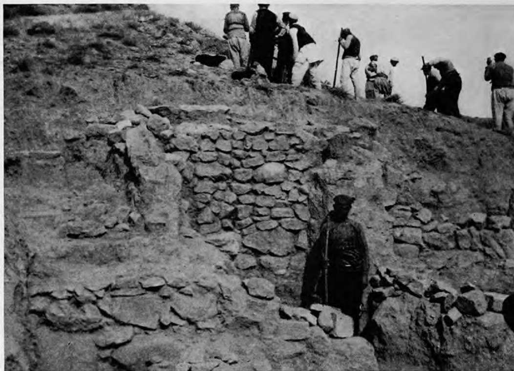
FIG. 81.—PLOT 23. VIEW OF WALLS; START OF WORK IN PLOT 25 (FROM WEST)
