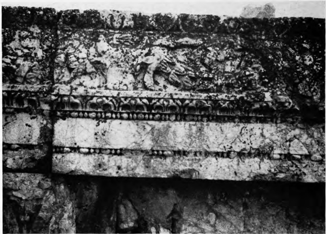
FIGS. 22 AND 23.—TERZILI HAMMAM. DETAILS OF FAÇADE OF ROMAN THERMAE
