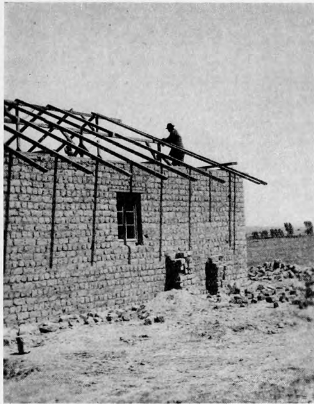
FIG. 50.—ROOFING THE HOUSE
