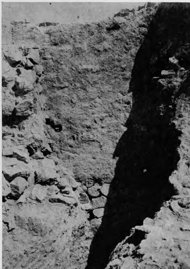
FIG. 177.—MAIN KERPICH WALL AT POINT SHOWN IN CROSS-SECTION NO. 1. STONE REVETMENT, REMOVED HERE, SHOWS AT EACH SIDE
