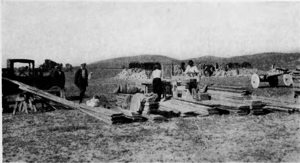
FIG. 49.—THE CONSTRUCTION OF THE CAMP
