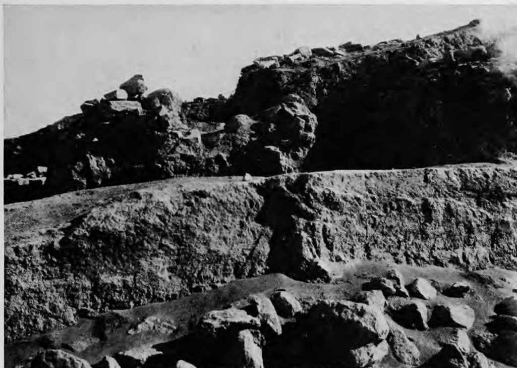
FIG. 175.—MAIN KERPICH WALL BETWEEN TOWER b AND CROSS-SECTION No. 3
