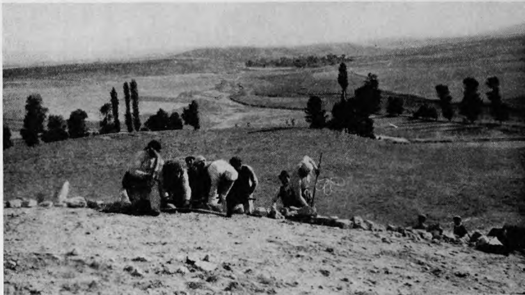
FIG. 110.—PLOT 33. START OF WORK (FROM NORTH)
