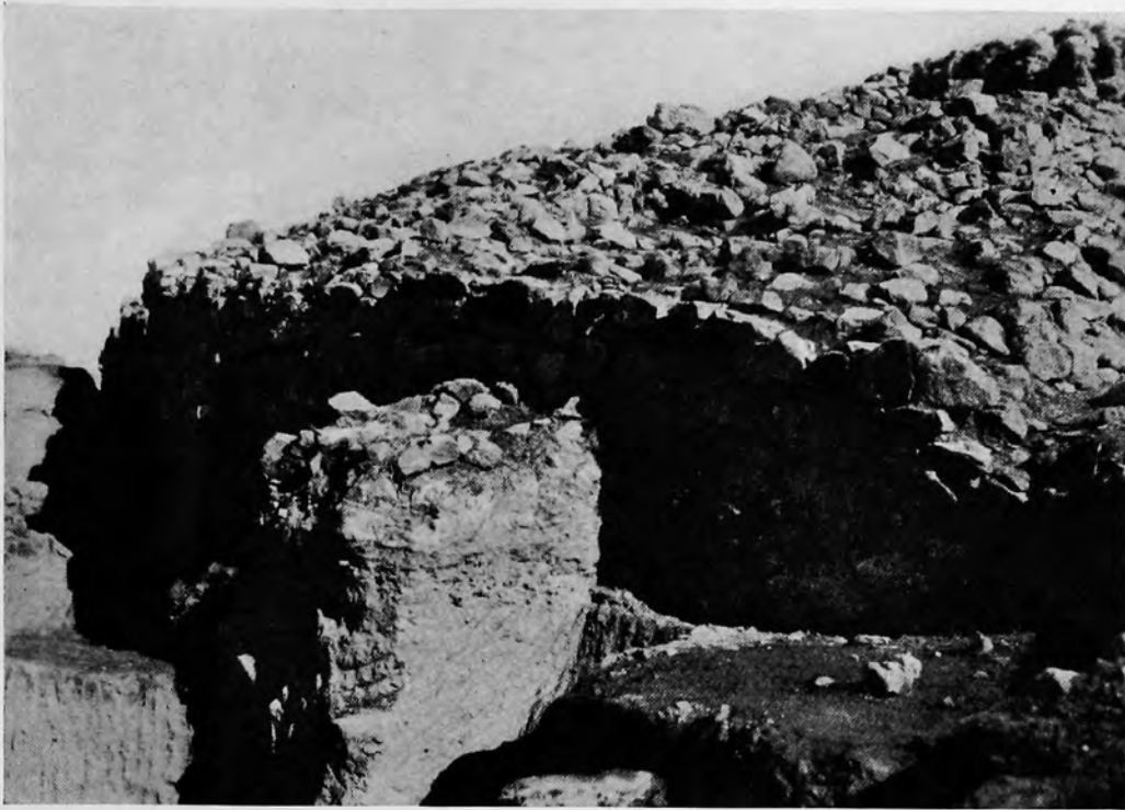
FIG. 182.—THE CITADEL WALL. BEND IN UNIT A
