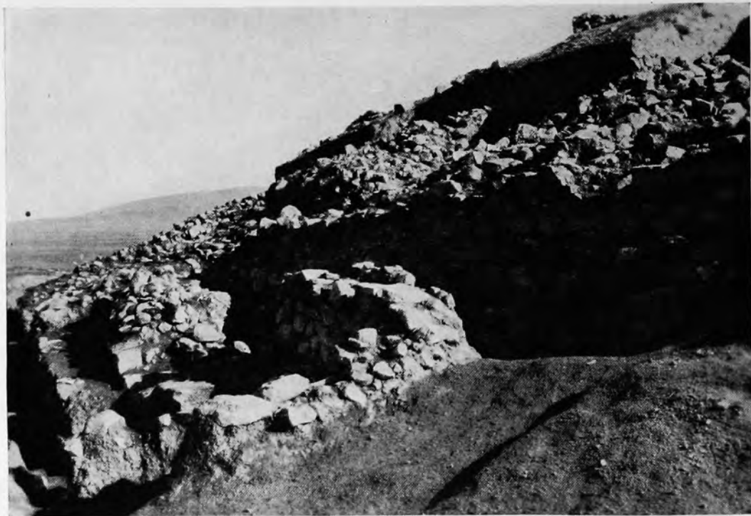
FIG. 185.—THE CITADEL WALL. UNITS A AND B NEAR CROSS-SECTION NO. II
