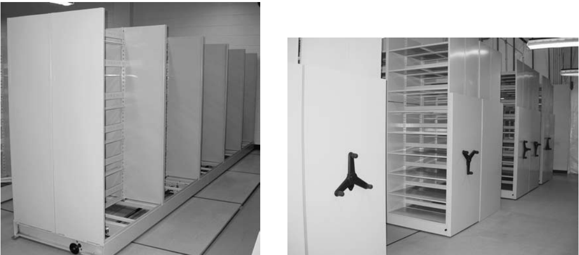
Figure 2. After the installation of the collapsible archival shelving
