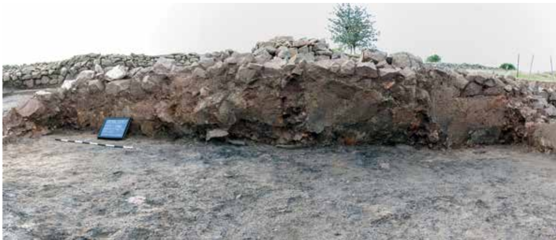
Figure 12. Wall plaster on the northern wall of Room 5 in Trench 31. Note the slots for wooden vertical beams spaced roughly every meter
