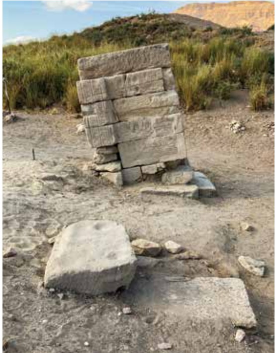
Figure 8. Claudius Gate prior to dismantling. Photo by Frank Hemholz.
