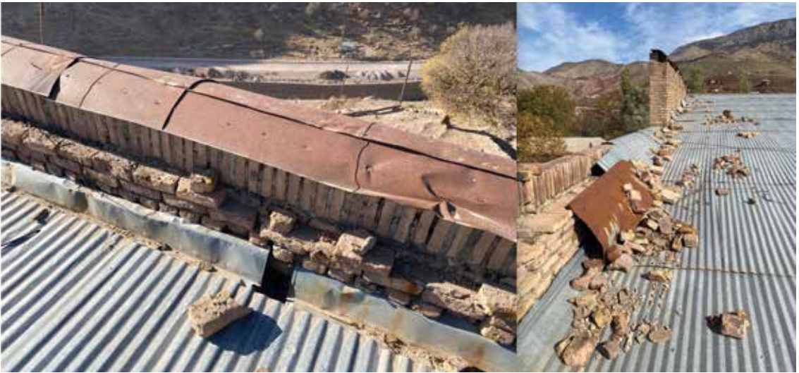
Figure 10. Current condition of the existing metal roof, brick parapet, and walls of the Langar Ota mosque. Preventing further water damage to the structure is the top priority. The leaking metal roof will be removed and replaced with a thicker-gauge, corrugated metal roof with waterproof sealing and improved rain gutters.
