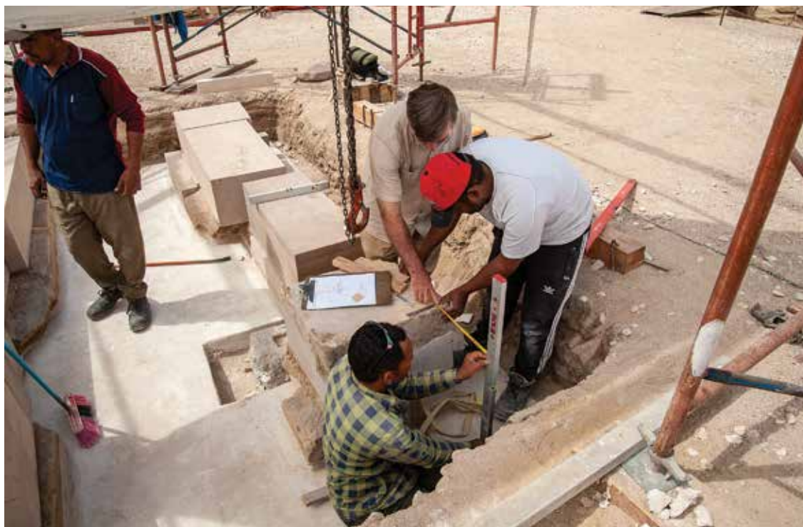
Figure 9. Stonemasonry team reerecting blocks of the Tahrqa Gate. Photo by Mohamed Abo el-Makarem.
