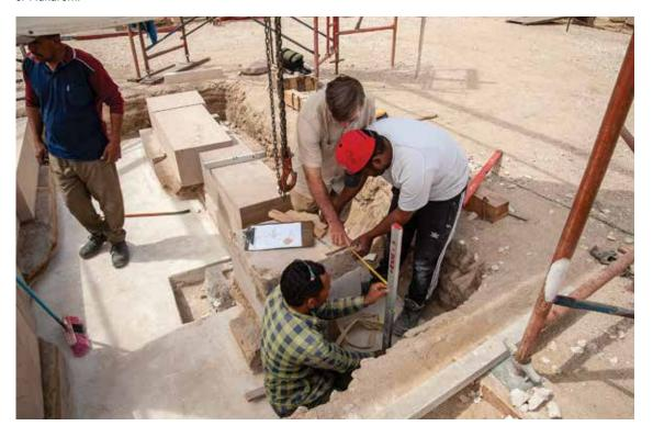
Figure 9. Stonemasonry team reerecting blocks of the Taharqa Gate. Photo by Mohamed Abo el-Makarem.
