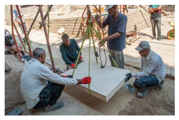
Figure 6. Stonemasonry team installing new sandstone paving block in the north sector of the Ramesses III mortuary temple. Photo by Frank Helmholz.
