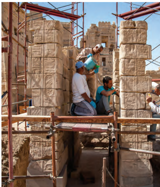
Figure 5. Stonemasonry team rebuilding the jambs of the Taharqa Gate. Photo by Frank Helmholz.
