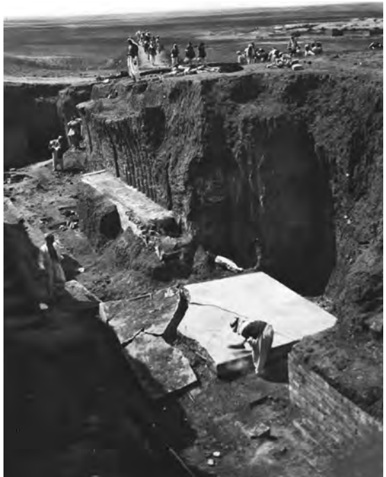
Figure 8. The excavation of the threshold of the entrance to the Sin Temple at Khorsabad, with the glazed-brick facades visible on each side (P. 21764/N. 11660).
