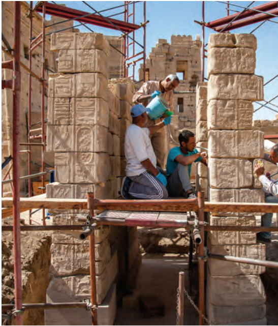
Figure 5. Stonemasonry team rebuilding the jambs of the Taharqa Gate. Photo by Frank Helmholz.
