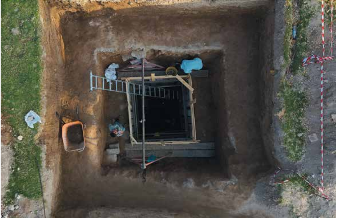
Figure 5. Stepping and shoring in trench SH10 to safely reach 8.4 m below ground surface.
