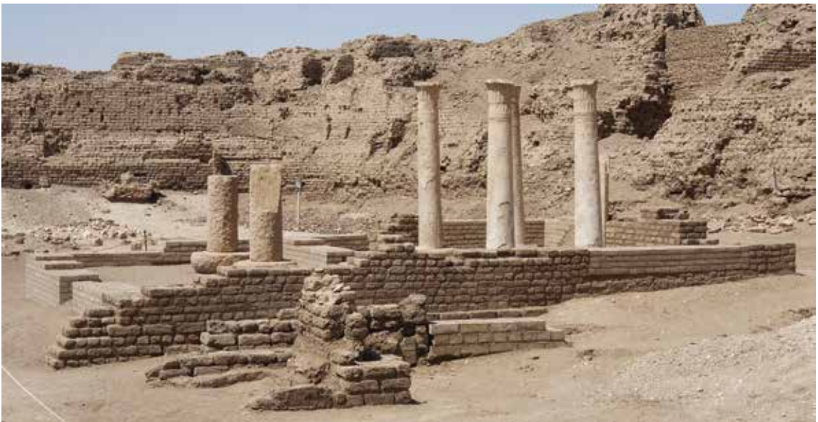
Figure 17. Butehamun House restoration finished, April 2017 (photo: Ray Johnson)
