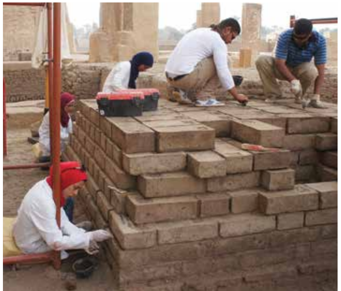
Figure 14. Brick wall restoration going up, Medinet Habu (photo: Ray Johnson)
