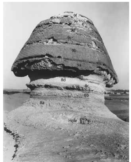
Figure 8. The back of the Sphinx head. Photo taken Sept. 25, 1925, before Baraize filled in the recesses and neck with ceramic bricks, limestone, and cement; view to the east (photo: Archive Lacau C I 006)
