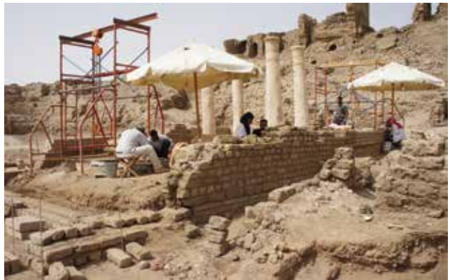
Figure 16. Butehamun House restoration work (photo: Ray Johnson)
