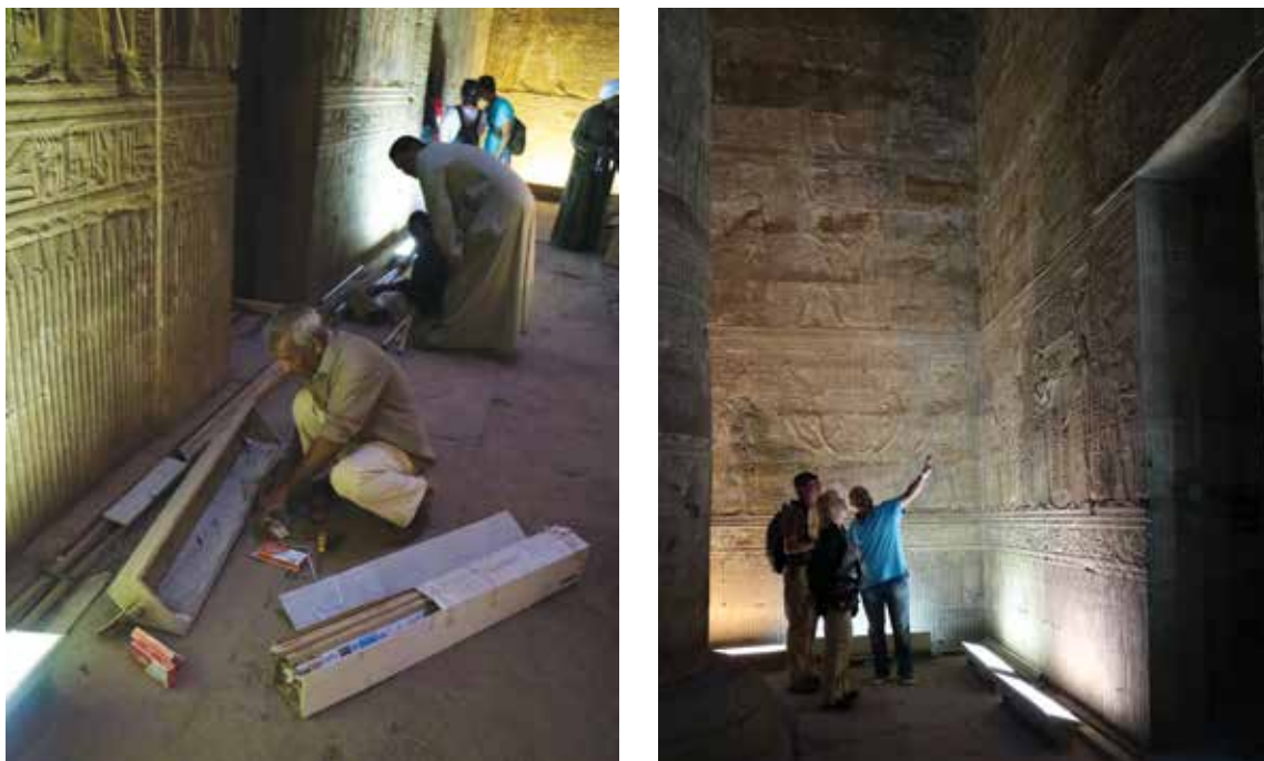
Figure 12a-b. Installation of new lights in the temple of Edfu
