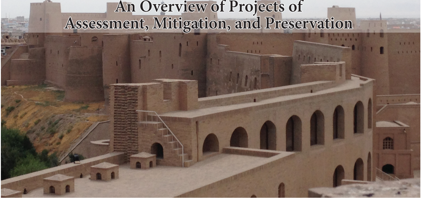
Qalat Ihtiyaraddin Citadel in Herat – restored by the Agha Khan Trust for Culture, with funding from the US Department of State. Photograph by Gil Stein.
