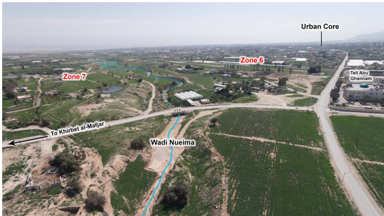
Figure 52: Aerial photo showing the Wadi Nueima dividing Khirbet al-Mafjar (Zone 7) from the rest of the Jericho plain (looking east; taken by author)
