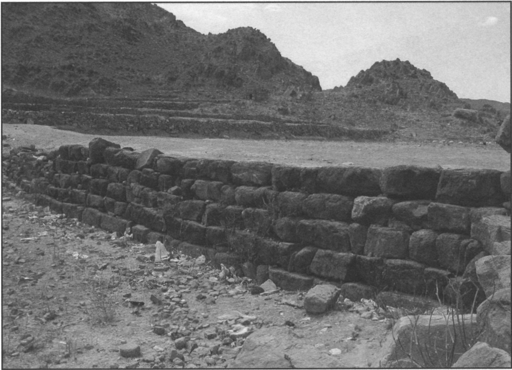
Figure 3. Cross-valley wall or dam at Qifl al-Shalalah. Photograph by Joseph Daniels
