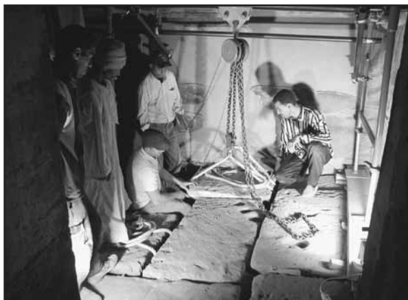
Figure 6. Dany and Chicago House temple workmen placing the final floor block in the "naos room" sanctuary, small Amun temple. Medinet Habu, Egypt. Photograph by Ray Johnson
