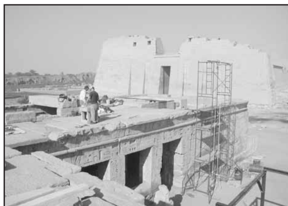
Figure 5. Dany and Ali working on the small Amun temple bark sanctuary roof. Medinet Habu, Egypt. Photograph by Ray Johnson
