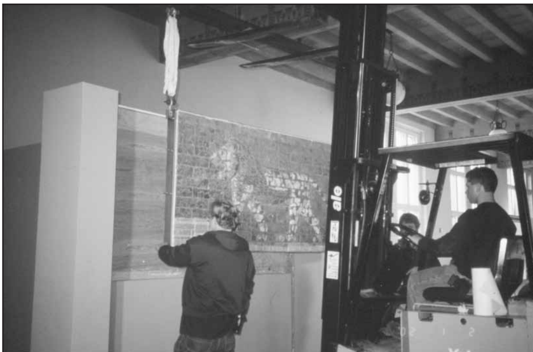
Figure 3. Ken Clesson and Robert Pizur of Belding/Walbridge installing one of the Babylon lions
