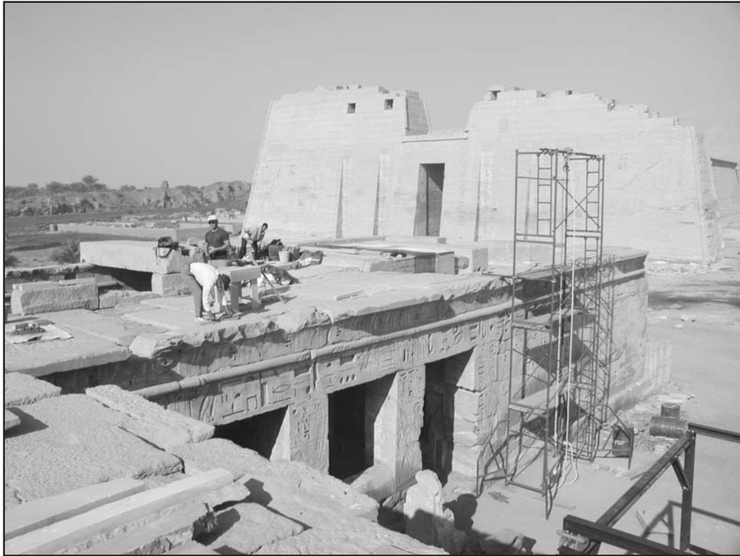
Figure 6. Dany Roy and Chicago House workmen doing restoration work on the roof of the small Amun temple, Medinet Habu. Digital photograph by Ray Johnson
