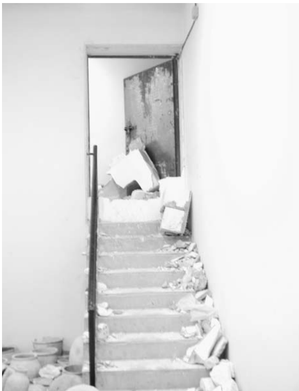
Iron door to basement storage and protective block wall penetrated by looters between April 10 and 11. Iraq National Museum
