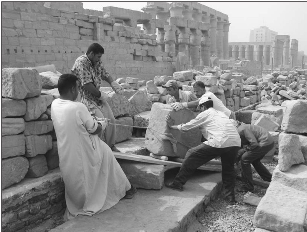
Figure 9. Chicago House workmen and SCA inspector moving blocks in the west area, Luxor Temple. Digital photograph by Ray Johnson
