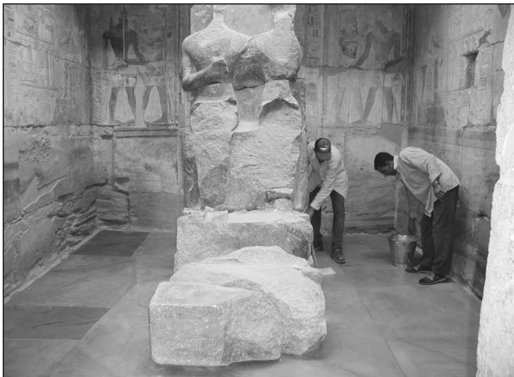
Figure 7. New sandstone floor and newly cleaned walls, front central sanctuary, small Amun temple, Medinet Habu. Digital photograph by Ray Johnson
