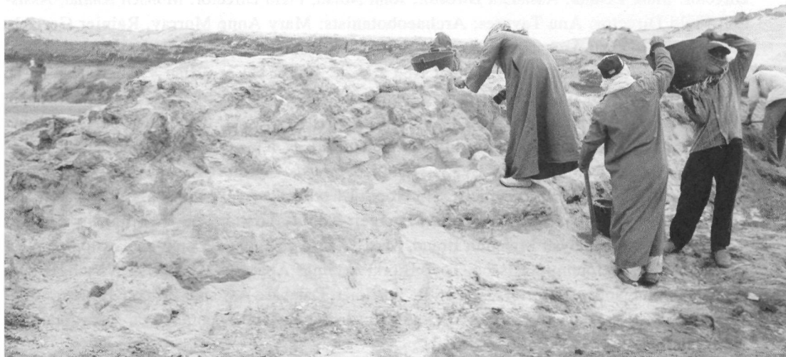
Figure 15. Workmen cleaning sand off Standing Wall, view to the southwest
