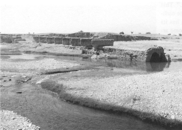
The siphon-bridge at Jundi-Shapur
