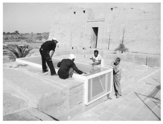
Installation of aluminum and frosted glass skylight over "dyad room," small Amun temple, Medinet Habu. Photograph by Ray Johnson
