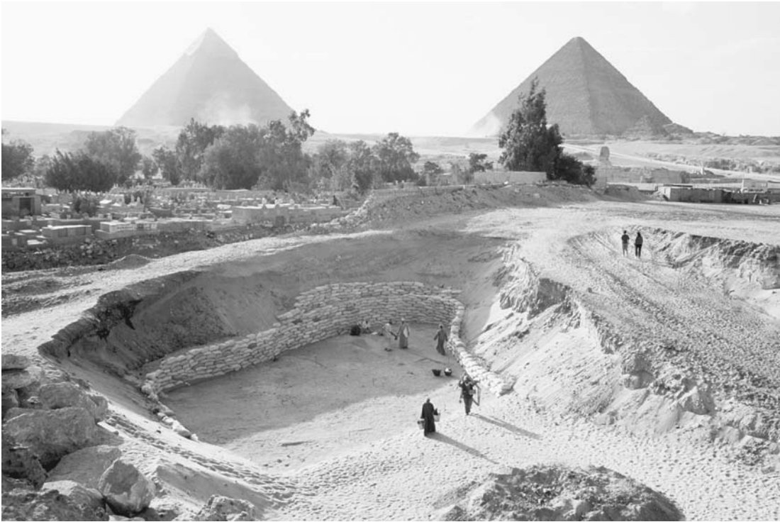
Figure 3. The clearing operation north of the Wall of the Crow Gate (WCGN), looking from the top of the wall to the northwest
