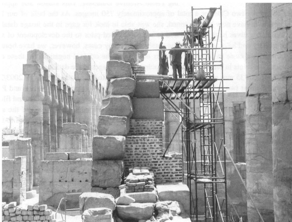
Figure 12. Brick buttress with sandstone veneer built against projecting eastern wall section of the Colonnade Hall, Luxor Temple, view from the north. Hassan Yousef Aly, Dany Roy, Saber Ahmed Taya, and Ali Mahmoud. Photo by Ray Johnson
