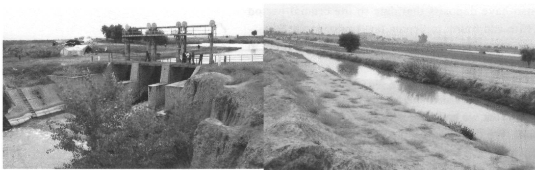
Figure 3. Left: Ojirub Dam; right: Khalaf irrigation canal, west of KS-004
