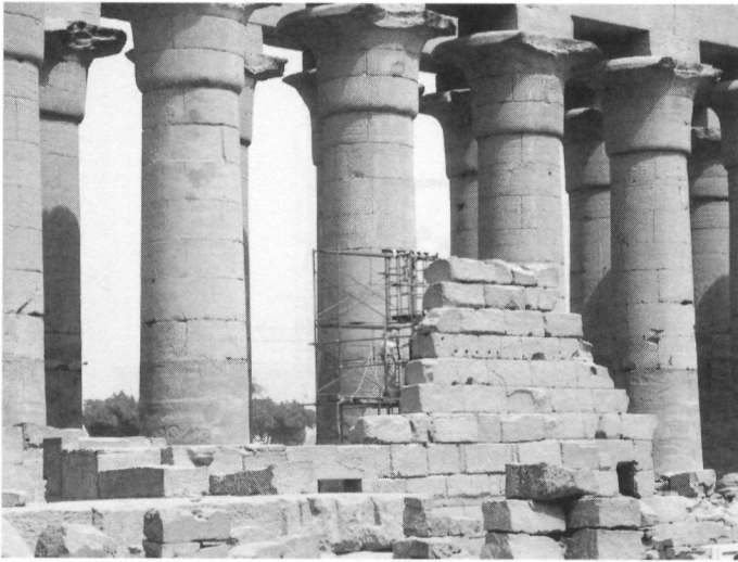
Figure 10. Projecting eastern wall section of the Colonnade Hall, Luxor Temple, view from the east. Photo by Ray Johnson
