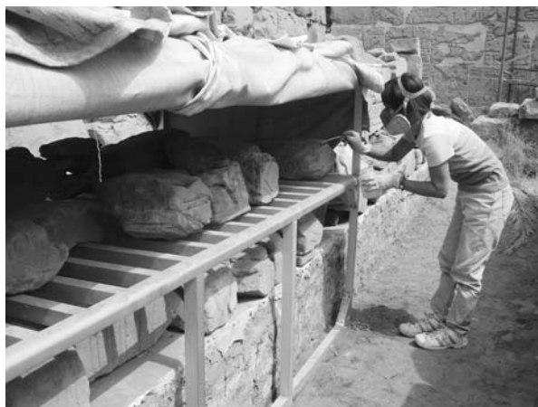
Hiroko Kariya doing emergency treatment of deteriorating decorated sandstone wall fragments. Northern blockyard treatment area, Luxor Temple. Photo by Ray Johnson
