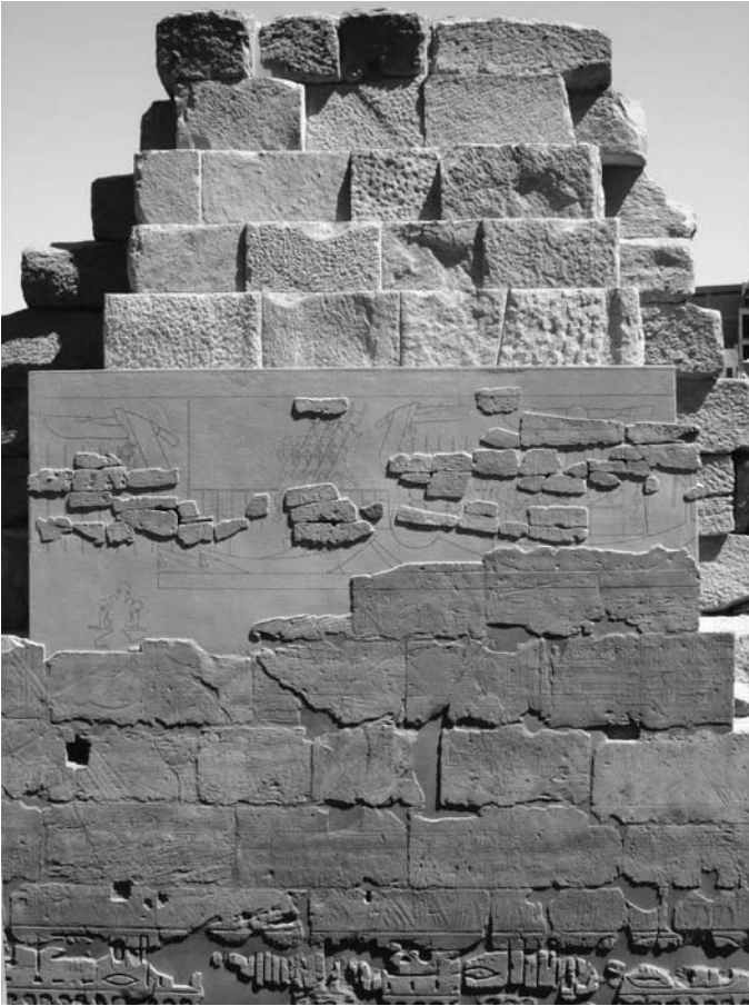
Stabilized and restored eastern wall section of the Colonnade Hall, Luxor Temple, with restoration drawing; view from the west. Photo by Ray Johnson
